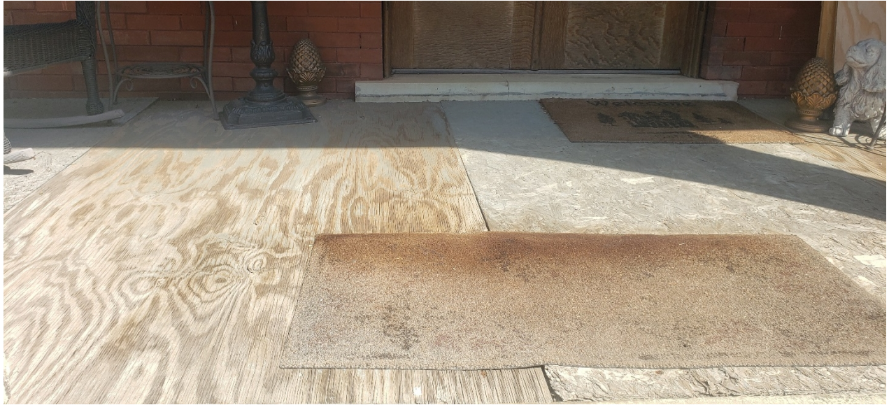
Attachment 1: Images of area where work is to be performed
