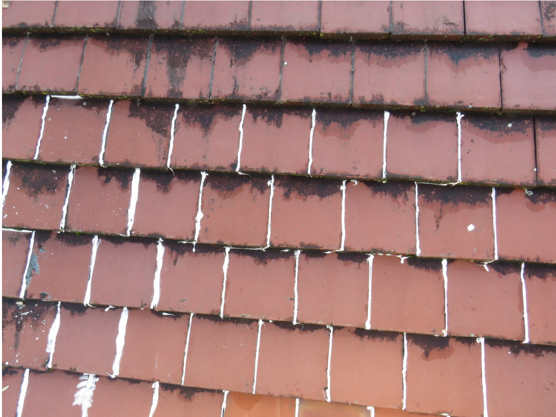
Attachment 1: Images of area where work is to be performed
