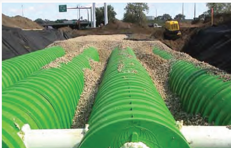
The lightweight and superior engineering of Triton Chambers made installation fast and easy.
