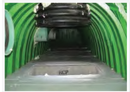
The Triton Main Header Row featured solid floors and an easily maintained sump dumpster.
