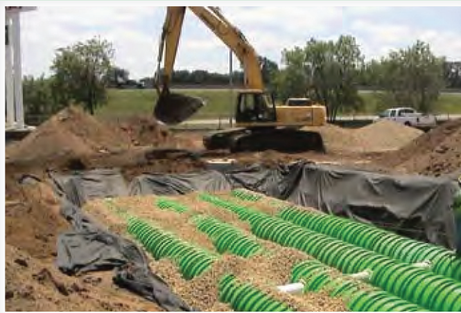
The Triton system is strong enough not to require a pavement layer allowing for construction equipment and customer traffic to move on and off the site during installation.
