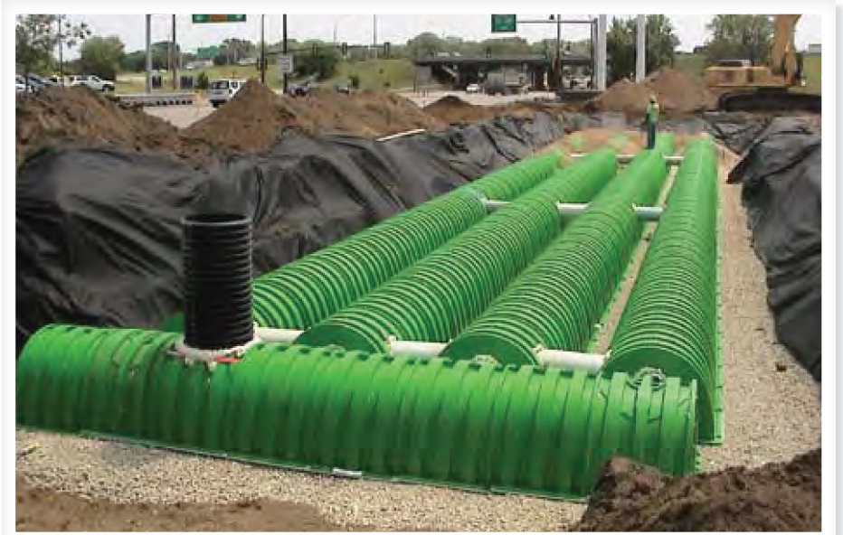
Phase one of Luther Brookdale Chevrolet underground storm water management system will have a storage volume of 11,000 cubic feet.
