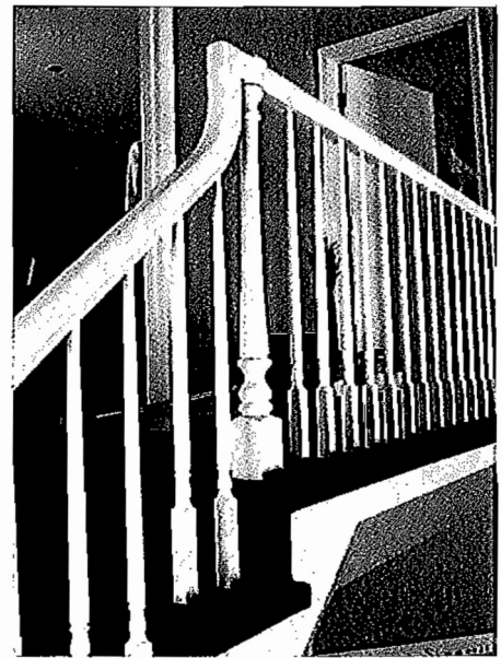
Transition from handrail to guard
