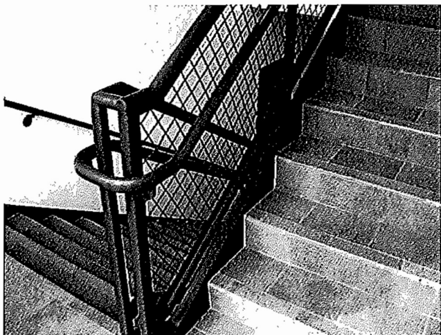
Interior exit stairway
