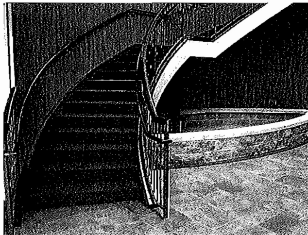
Exit access stairway
