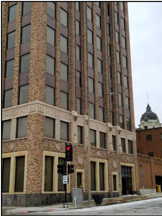
Figure 9 North elevation of the State Farm building.
