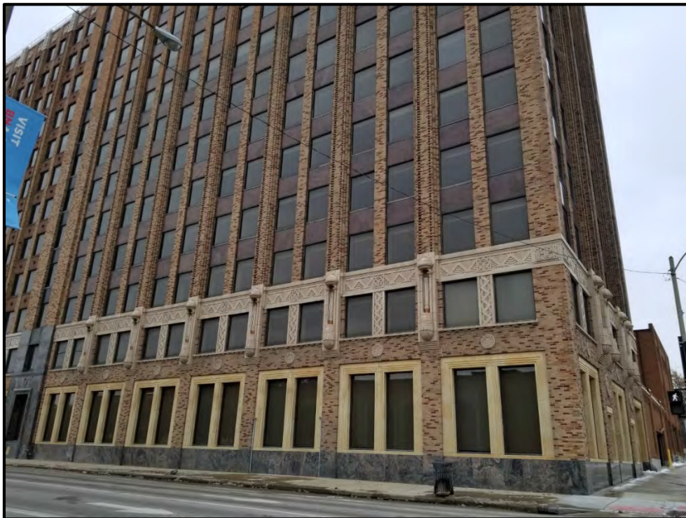
Figure 7 Northern portion of east elevation.
