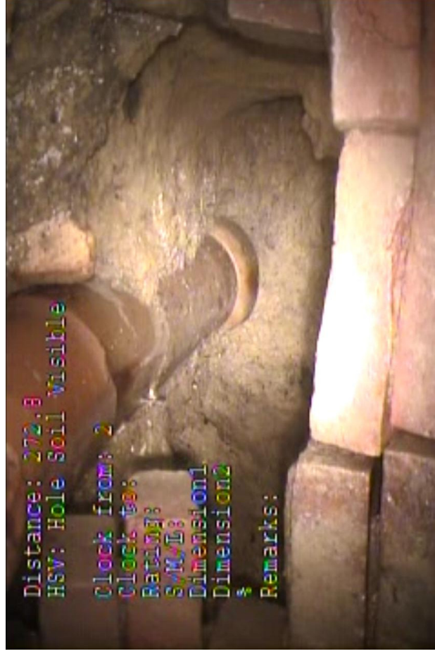
Holes in the Douglas Street Sewers filmed by CCTV
