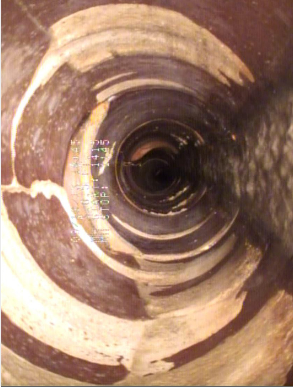
Clayton Street Sewer: Hinge cracking in clay sewer
