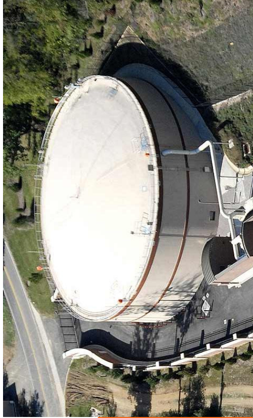
Wastewater storage facility, Knoxville, Tenn.
