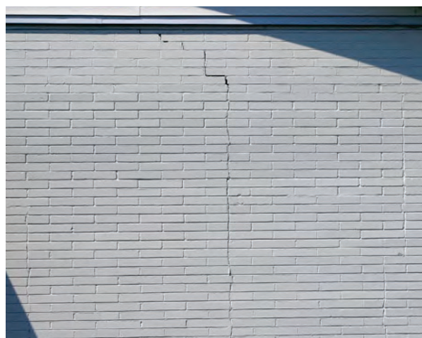
Right: Cracking in the exterior brick wall of this multi-tenant building. (1328 East Empire Street)
