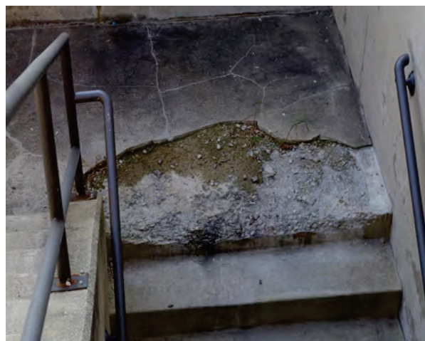
Right: The concrete of this stairwell at Bloomington High School is disintegrating.
