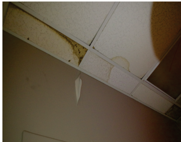
Right: Water damage to the interior ceiling tiles of the former Circuit City. (1500 East Empire Street, Suite 1A)
