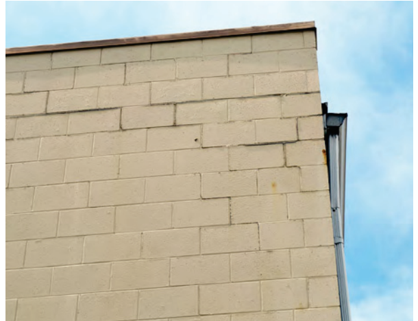
Left & Right: Step cracking in the exterior concrete block walls. (1215 Holiday Drive)
