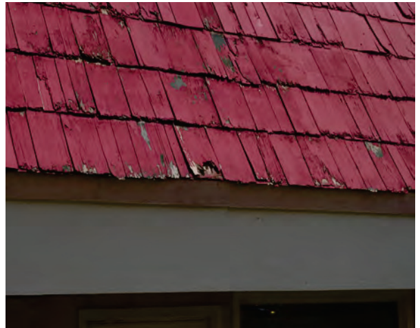
Left & Right: Deteriorated wood shakes on the roof of Kep's Country Kitchen. (506 IAA Drive)
