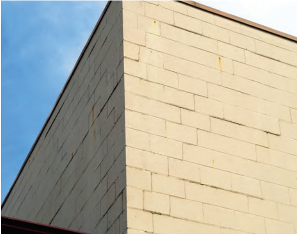
Left & Right: Step cracking in the exterior concrete block walls. (1215 Holiday Drive)
