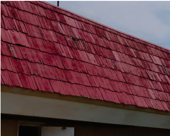
Left & Right: Deteriorated wood shakes on the roof of Kep's Country Kitchen. (506 IAA Drive)
