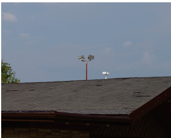
Left: The roof of Garden of Paradise is missing shingles. (1412 East Empire Street)
