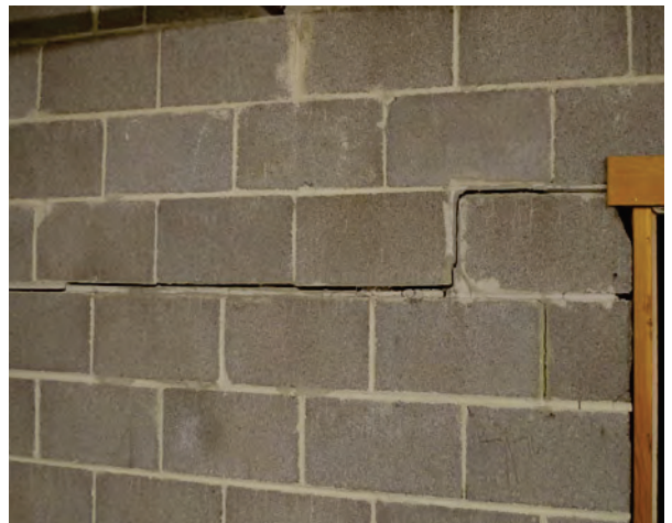
Left & Right: Cracking in the concrete block walls of the former K--Mart. (1608 East Empire Street)
