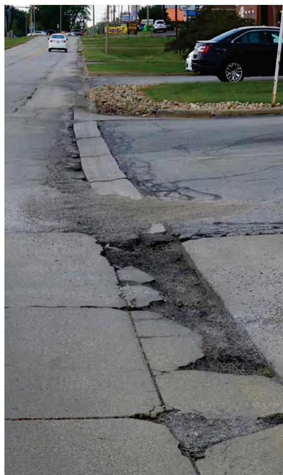
Left: The edge of pavement and the apron entering Colonial Plaza from the south are deteriorated.
