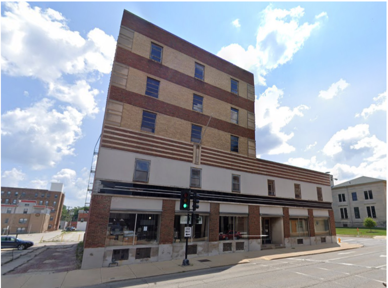
Above: The subject property
