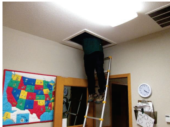
Checking attic insulation levels.
