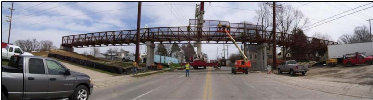
Figure 4.1. Constitution Trail bridge over Oakland Avenue.
