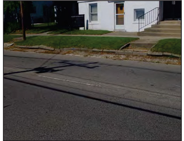
Right: The curbs along the west side of North Center Street are severely deteriorated.
