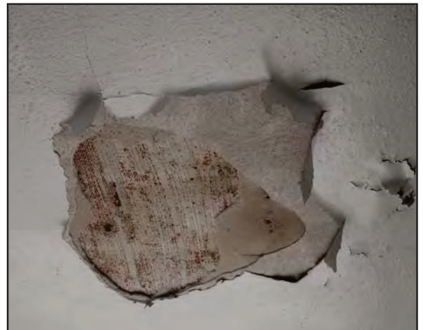
Left & Right: Water damage to the ceiling of the former Shell building.
