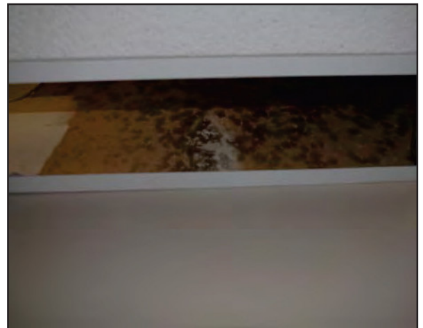
Left: Water damage around a window inside of the vacant dormitory
