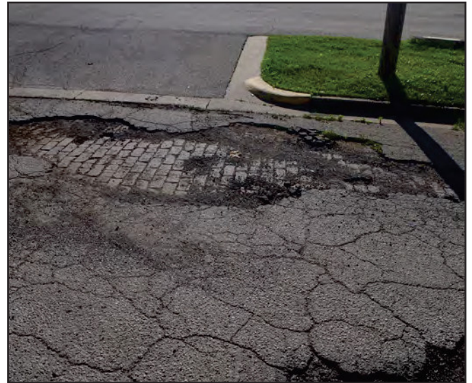
The asphalt pavement on North East Street, located on the 804 North East Street property, has disintegrated exposing the old brick street surface.
