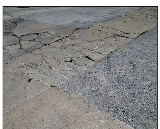
Left: The edge of the pavement along West Walnut Street is deteriorated. (Between North Main Street and North East Street)
