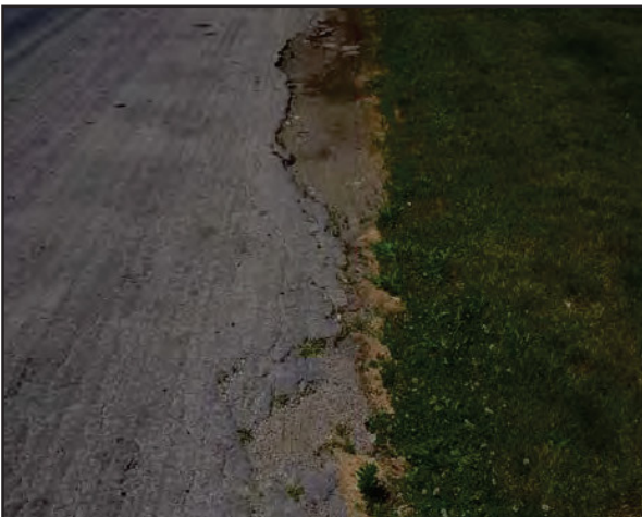
Left: The edge of the pavement along West Walnut Street is deteriorated. (Between North Main Street and North East Street)
