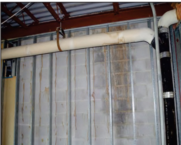
Left: Water running down the wall of the Creativity Center rusted the ceiling structure and stained the wall.
