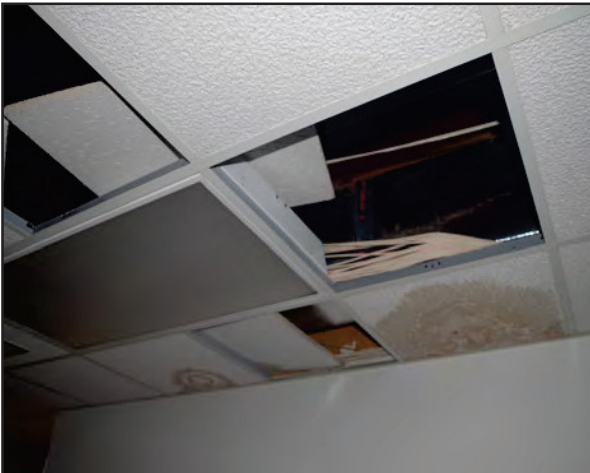
Left: Water damaged and collapsed ceiling tiles in the Creativity Center.
