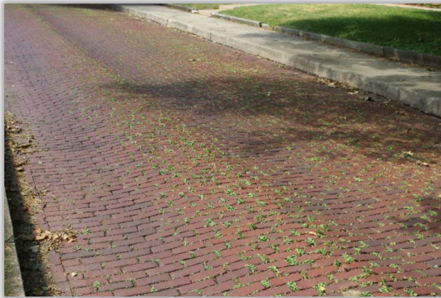
Figure 18: Effects of driving on vegetation between bricks
