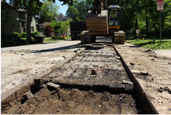
1. This process requires a backhoe with teeth in good condition or other, similar equipment.
