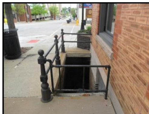
Figure 9: Sidewalk Vault Example
