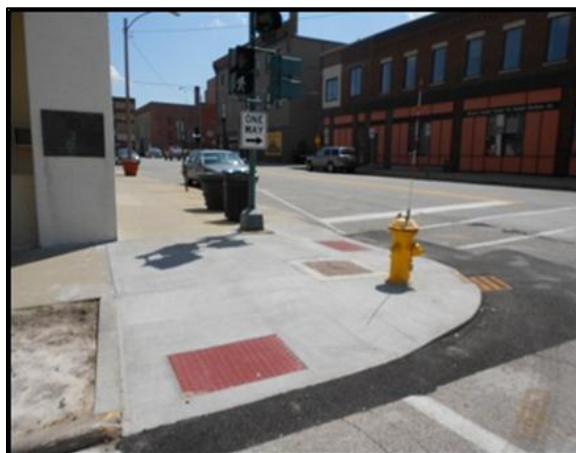
Figure 6: Example of Completed Inlet Repair Work
