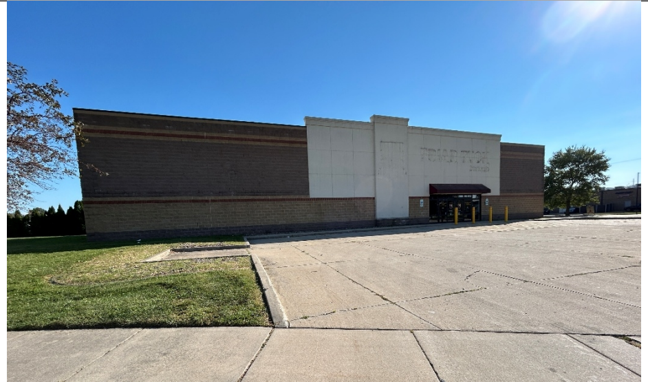
Figure 2. Looking south at subject property from Maloney Drive.
