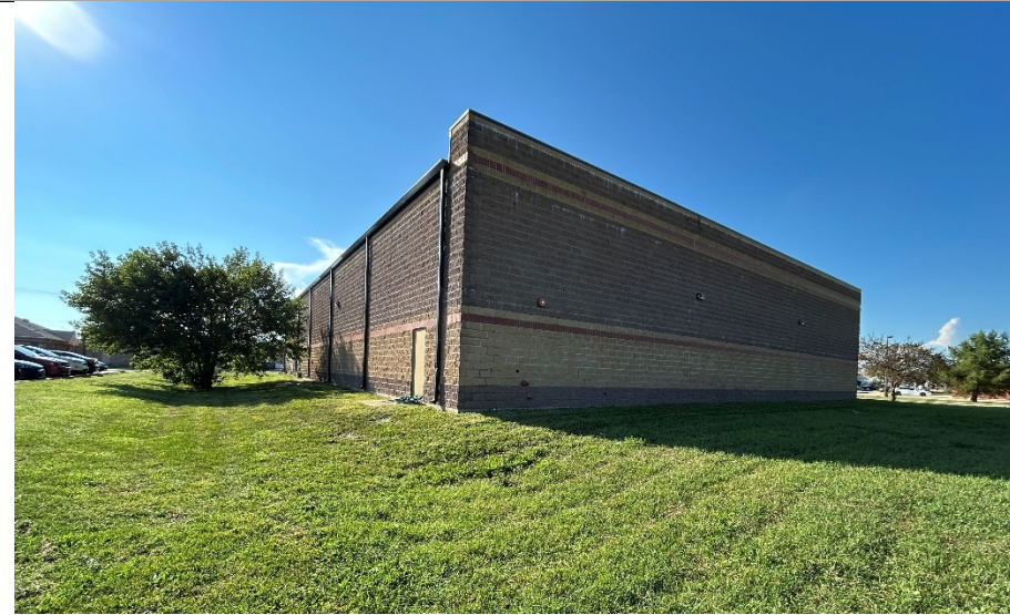
Figure 1. Looking northwest towards rear of subject property.
