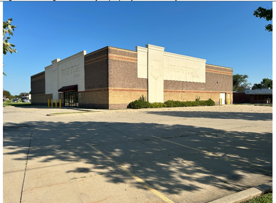
Figure 4. Looking southeast at subject property from parking lot.
