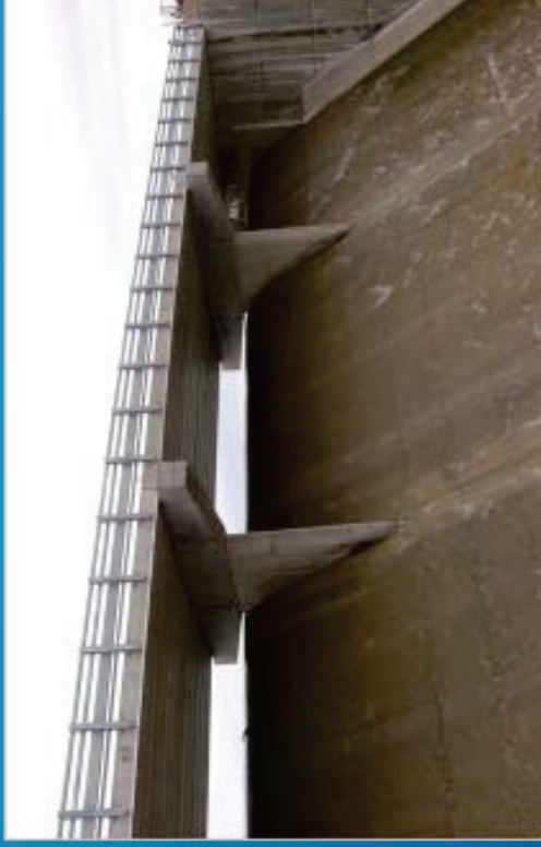
Evergreen Lake Dam Drain System Rehabilitation
