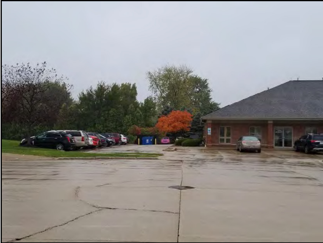
Figure 5 Front and side view of the office.
