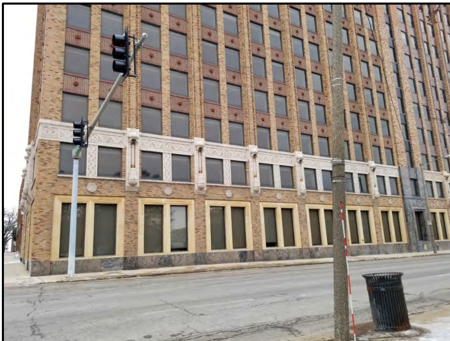
Figure 5 South portion of east elevation.
