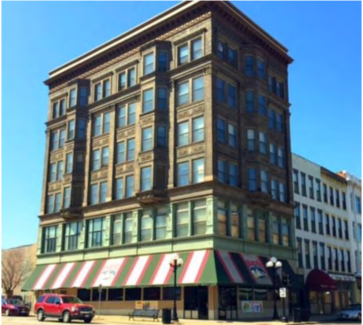
Livingston building exterior
