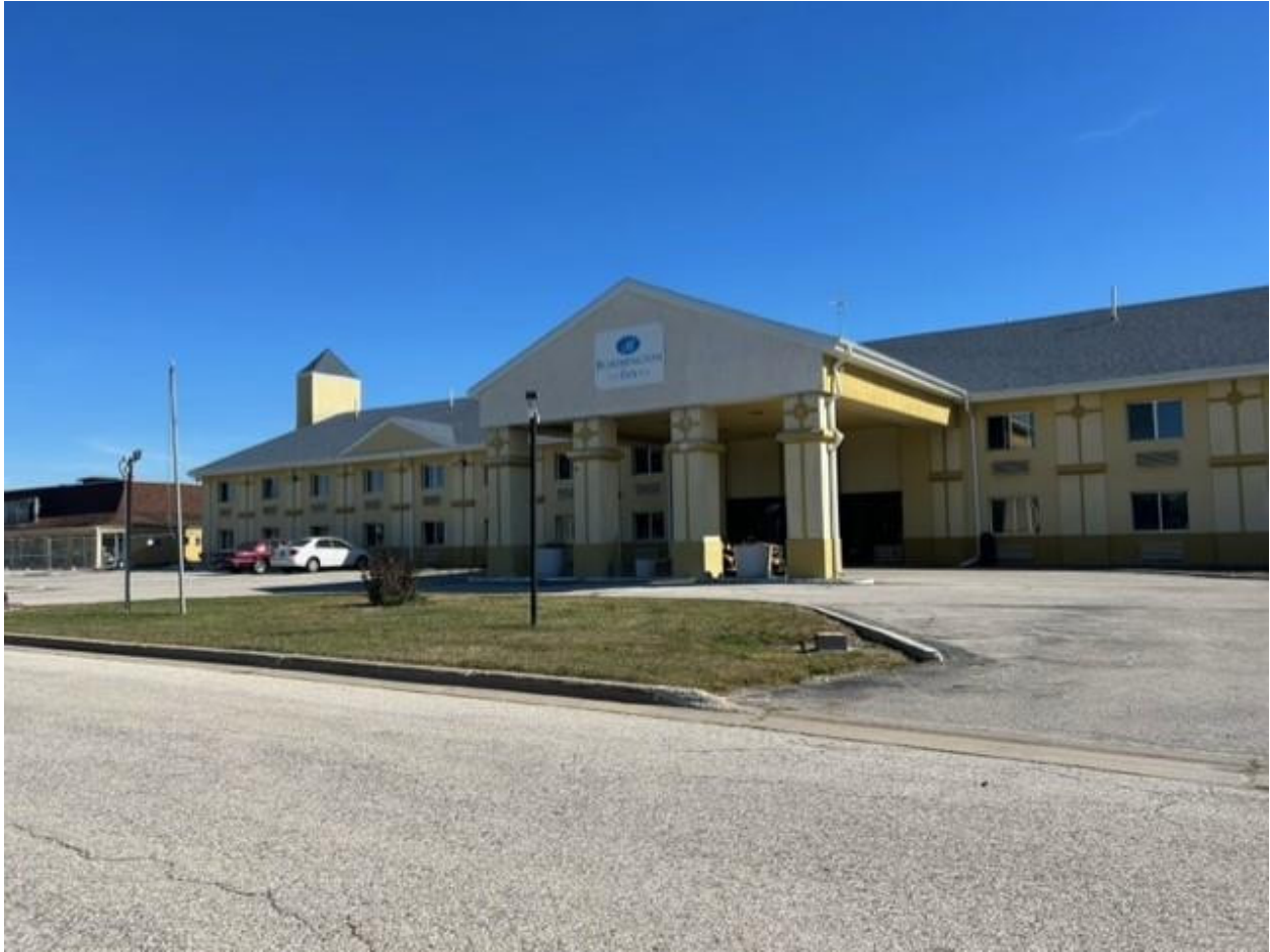
401 BROCK STREET – MAIN HOTEL BUILDING (NOT BEING DEMOLISHED)
