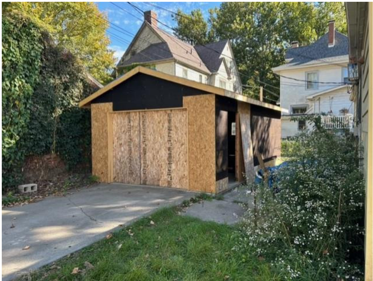
DETACHED GARAGE – 1103 N PARK STREET
