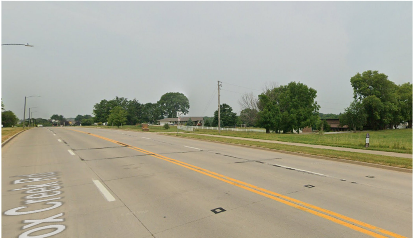
View West of Site
