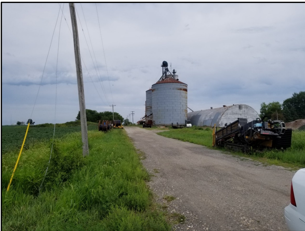
Figure 9 View looking east along the access road on the south boundary of subject property.
