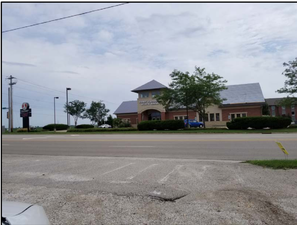
Figure 12 View of the bank on the southwest corner of the intersection.
