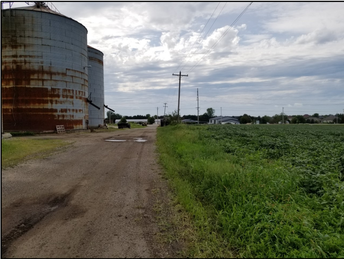
Figure 7 View along south access road showing the silos to the south of the property.
