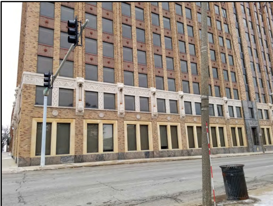
Figure 5 South portion of east elevation.
