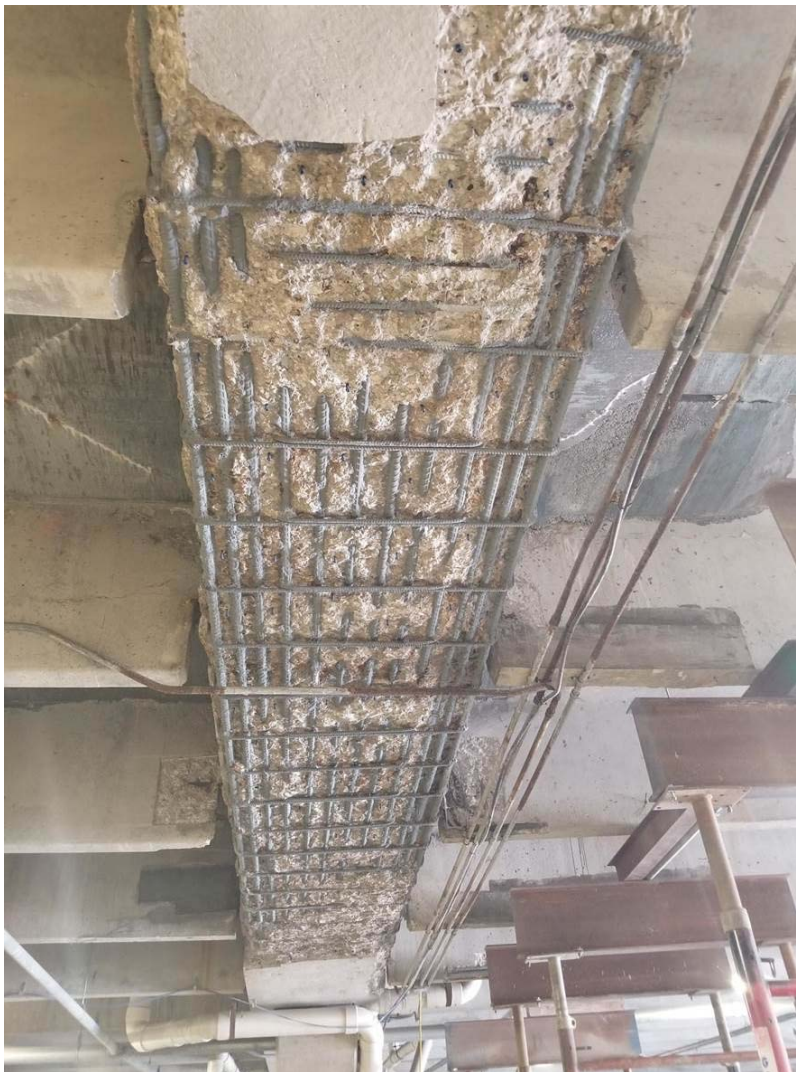
BEAM AFTER LOOSE CONCRETE REMOVAL
