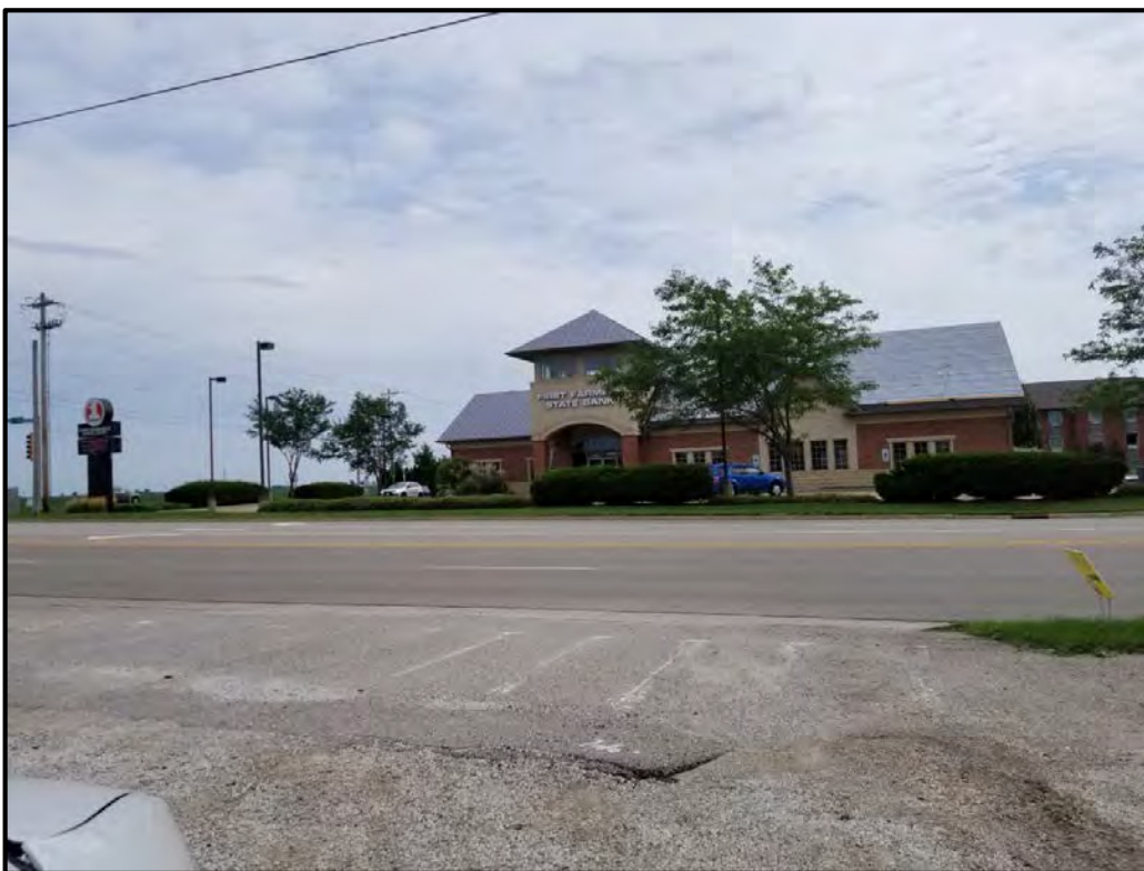
Figure 12 View of the bank on the southwest corner of the intersection.
