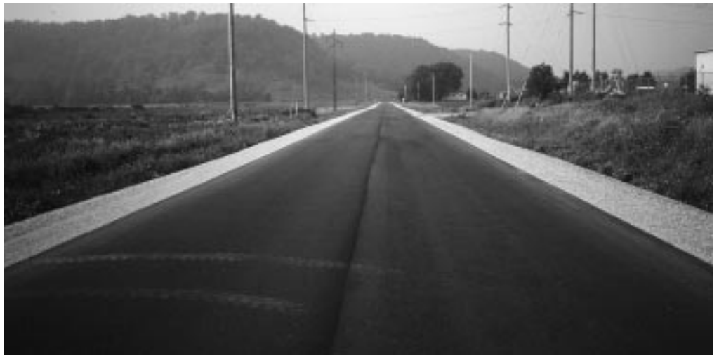
► RATING 9 Recent overlay, rural.
