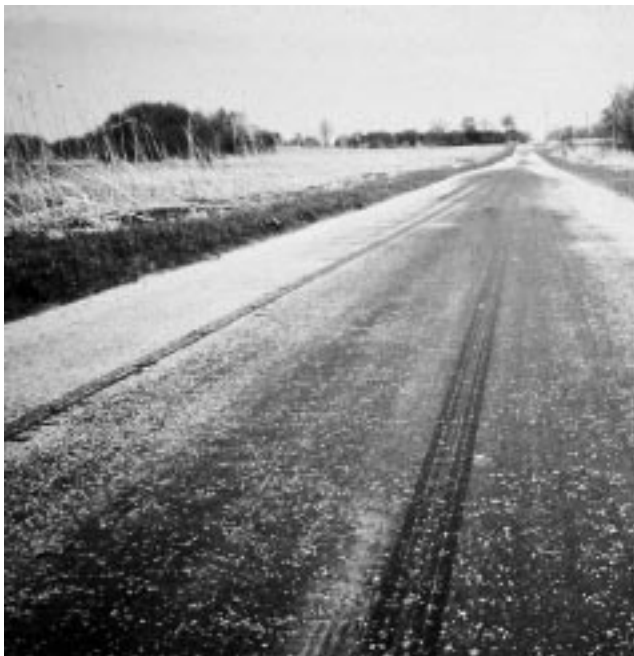
▼ Severe flushing.
