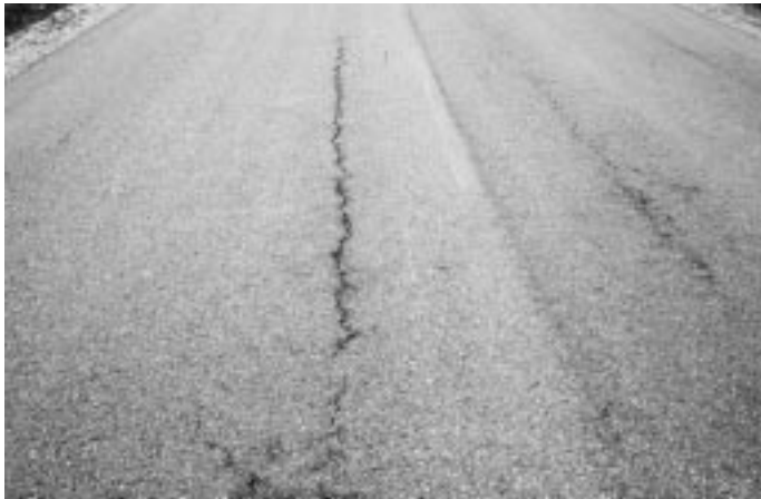
▶ First stage of wheelpath cracking caused by heavy traffic loads.
