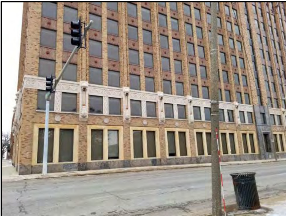
Figure 5 South portion of east elevation.
