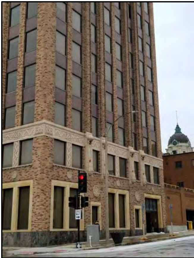
Figure 9 North elevation of the State Farm building.
