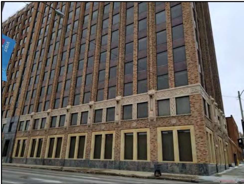
Figure 7 Northern portion of east elevation.
