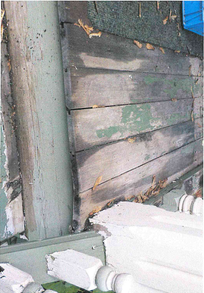
porch floor + spindles
