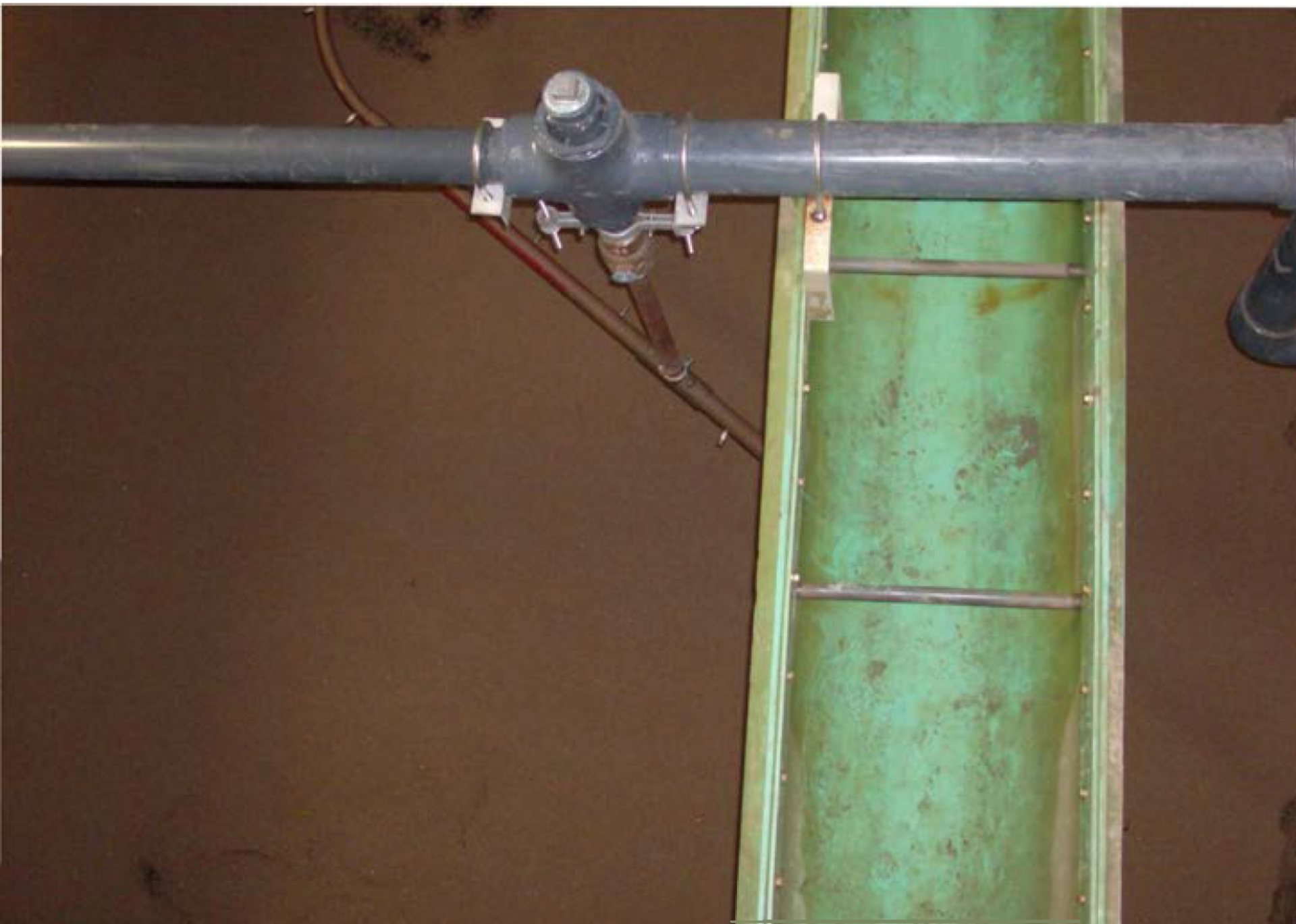
Sand media is added to the filter.
