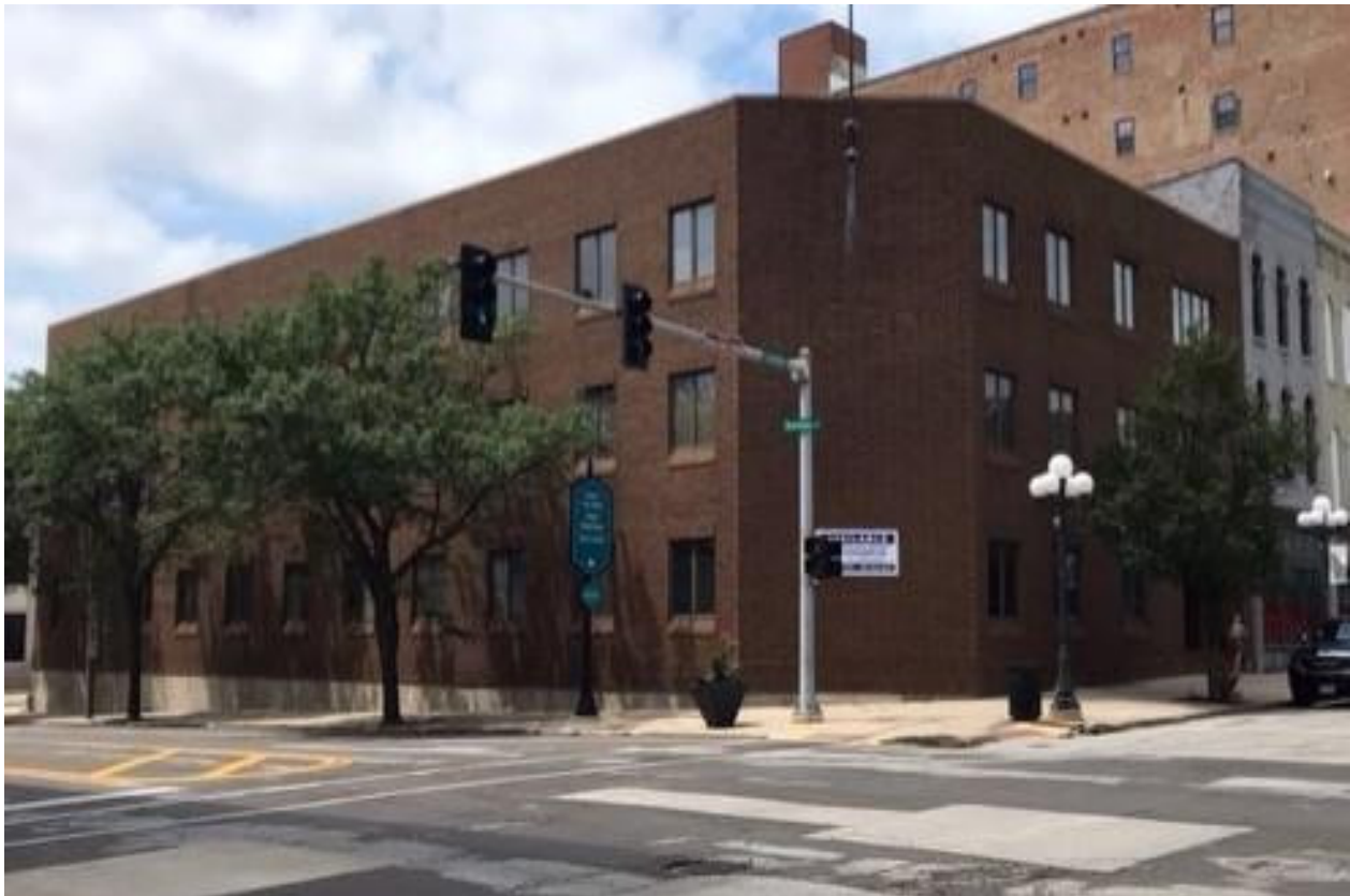
Above: The subject property at 202 Center Street.
