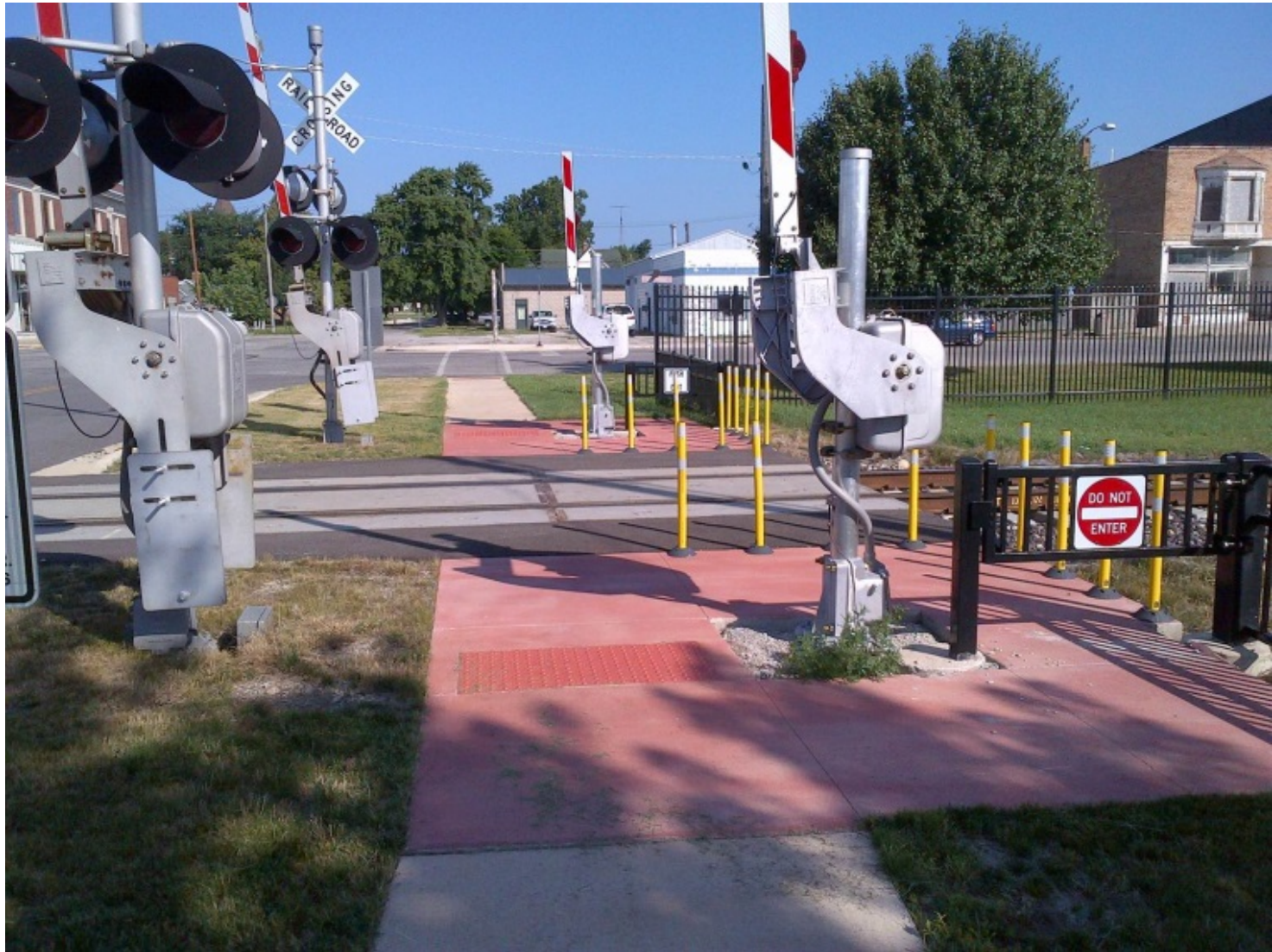
Typical pedestrian rail crossing installation
