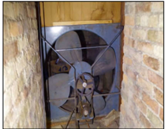
Right: A vent fan in the bell tower adjacent to the balcony lacks a safety screen.
