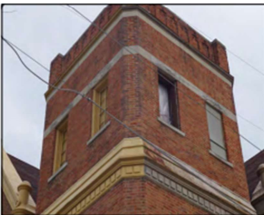
Left: A missing window in the church tower allows the weather and wildlife to enter into the structure.
