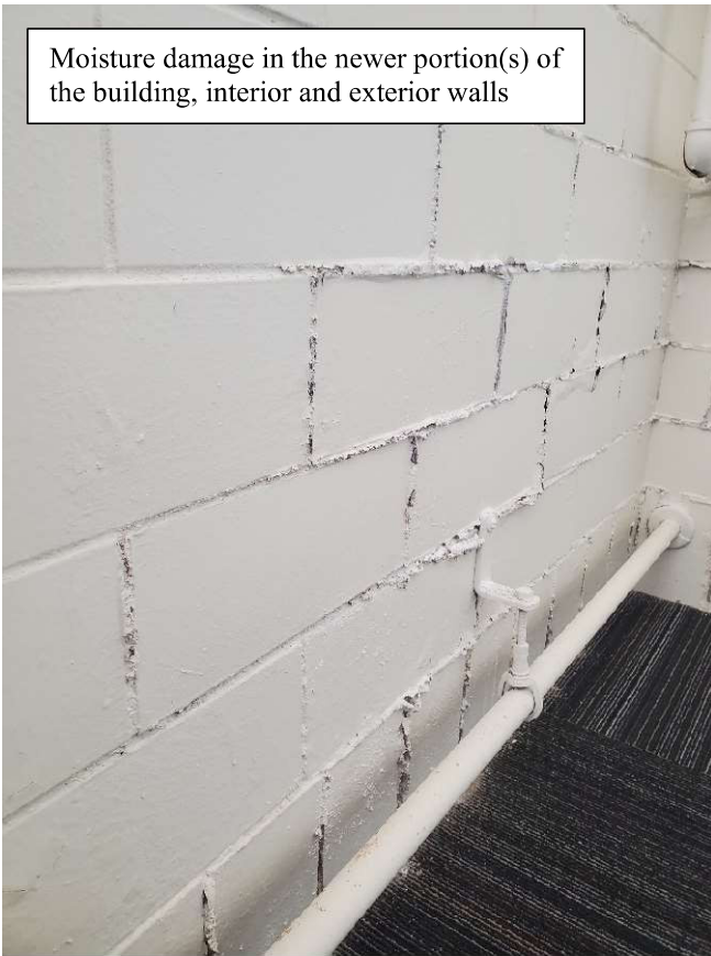
Continued moisture damage following roof repair/replacement
