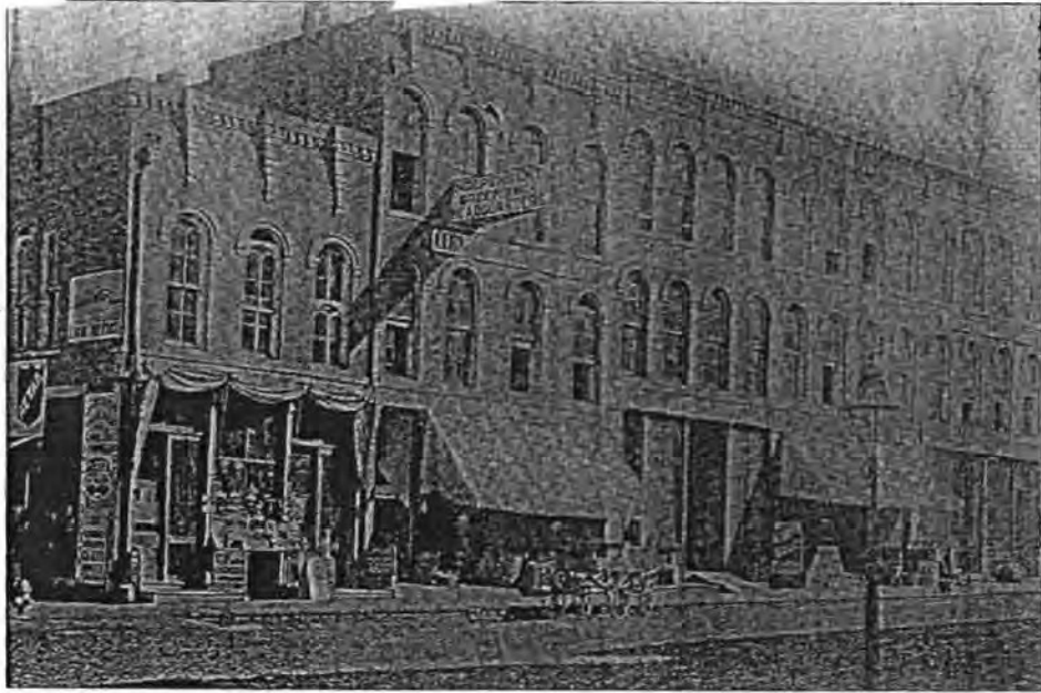
The Rounds Block, seen at right in this circa 1870 photograph, was a center of commerce and Bloomington social life from its inception in 1856-57. Parts of the building have been restored in recent years by Fred Wollrab.
