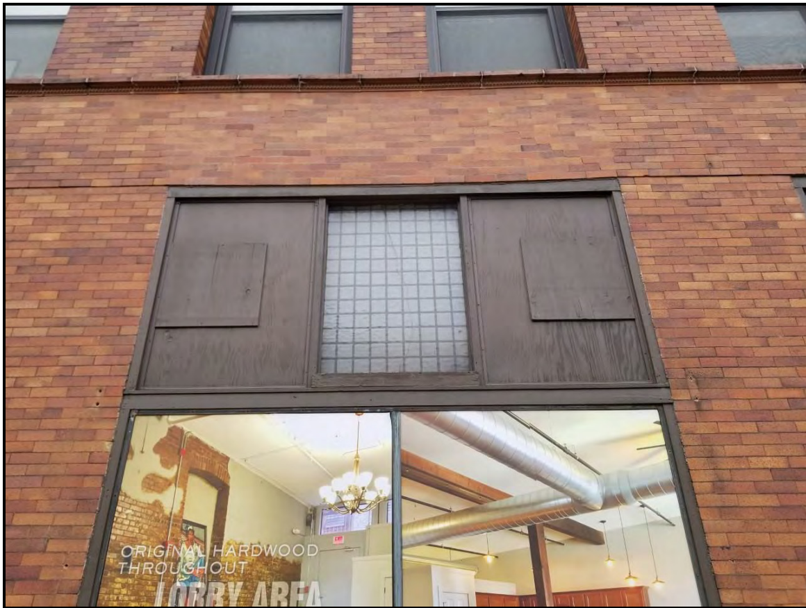
Figure 8 Transom windows on east elevation.
