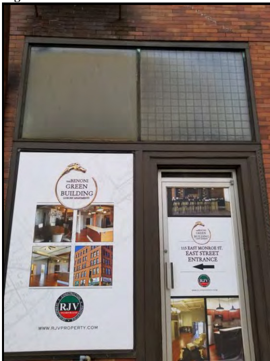
Figure 9 Door and transom windows on east elevation.
