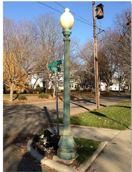
Figure 1 - An existing 10 foot decorative light pole and fixture on the corner of E. Grove Street and Harwood Place.
