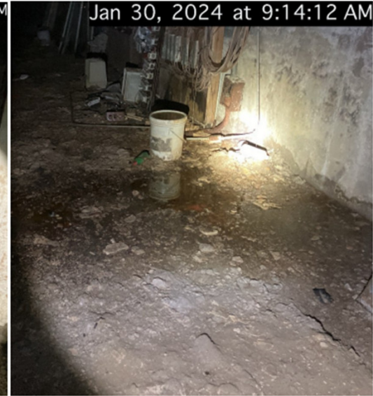
Standing water on the interior of the structure, foundation areas and other
