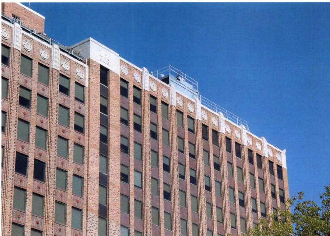
14. East elevation, north end parapet, looking northwest
