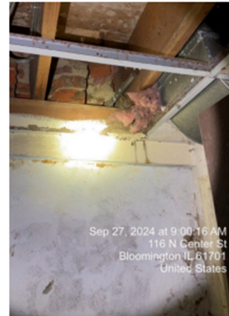
Beginning deterioration of metal components due to vacancy and lack of climate control
