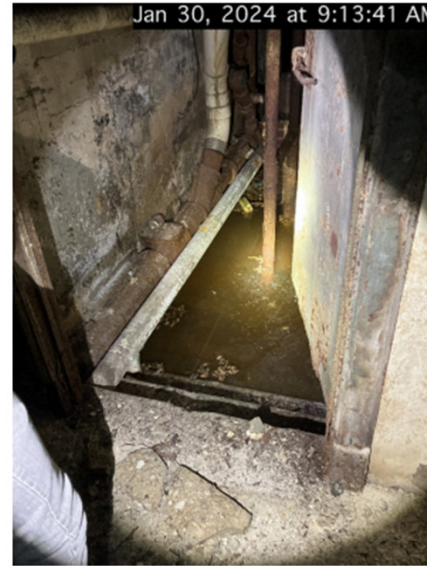
Standing water on the interior of the structure, foundation areas and other
