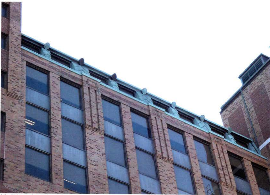
23. West elevation, detail of copper enclosure at top floor auditorium
