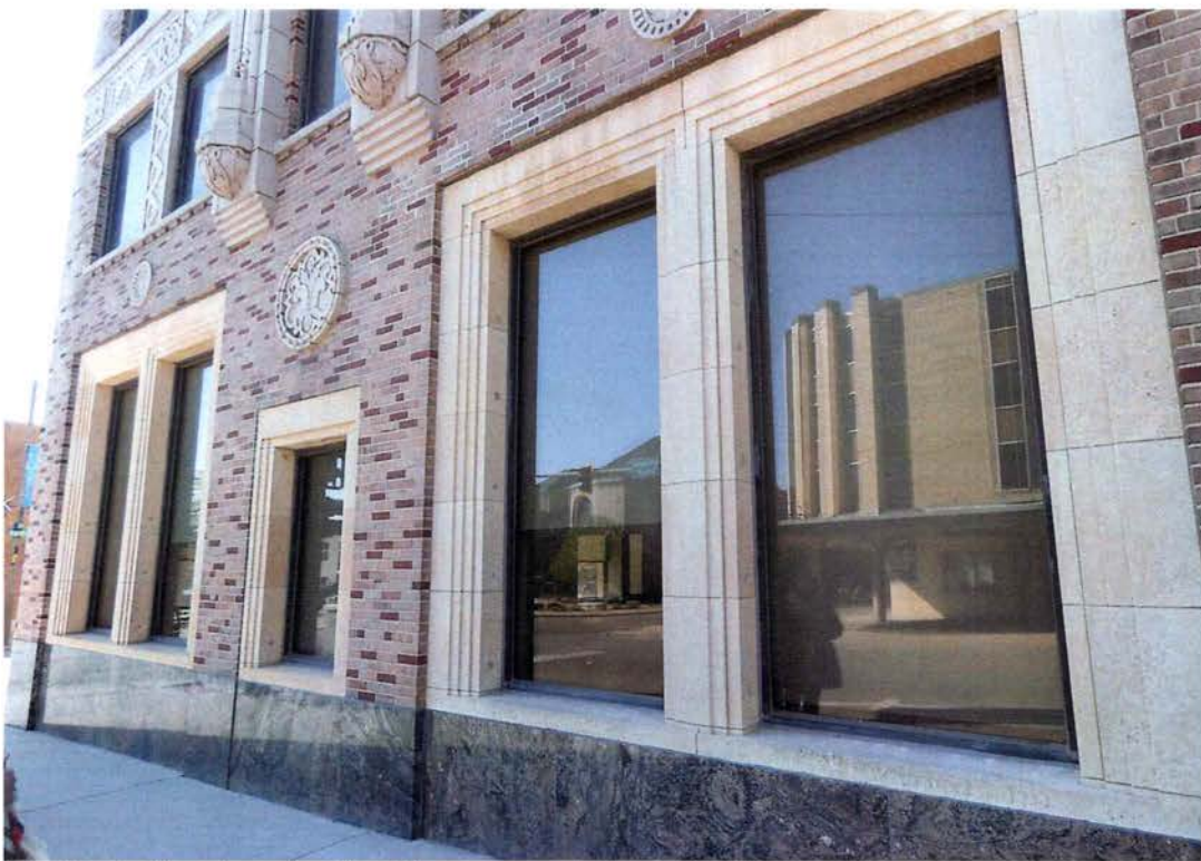
16. North elevation, detail of first-story windows, looking southeast
