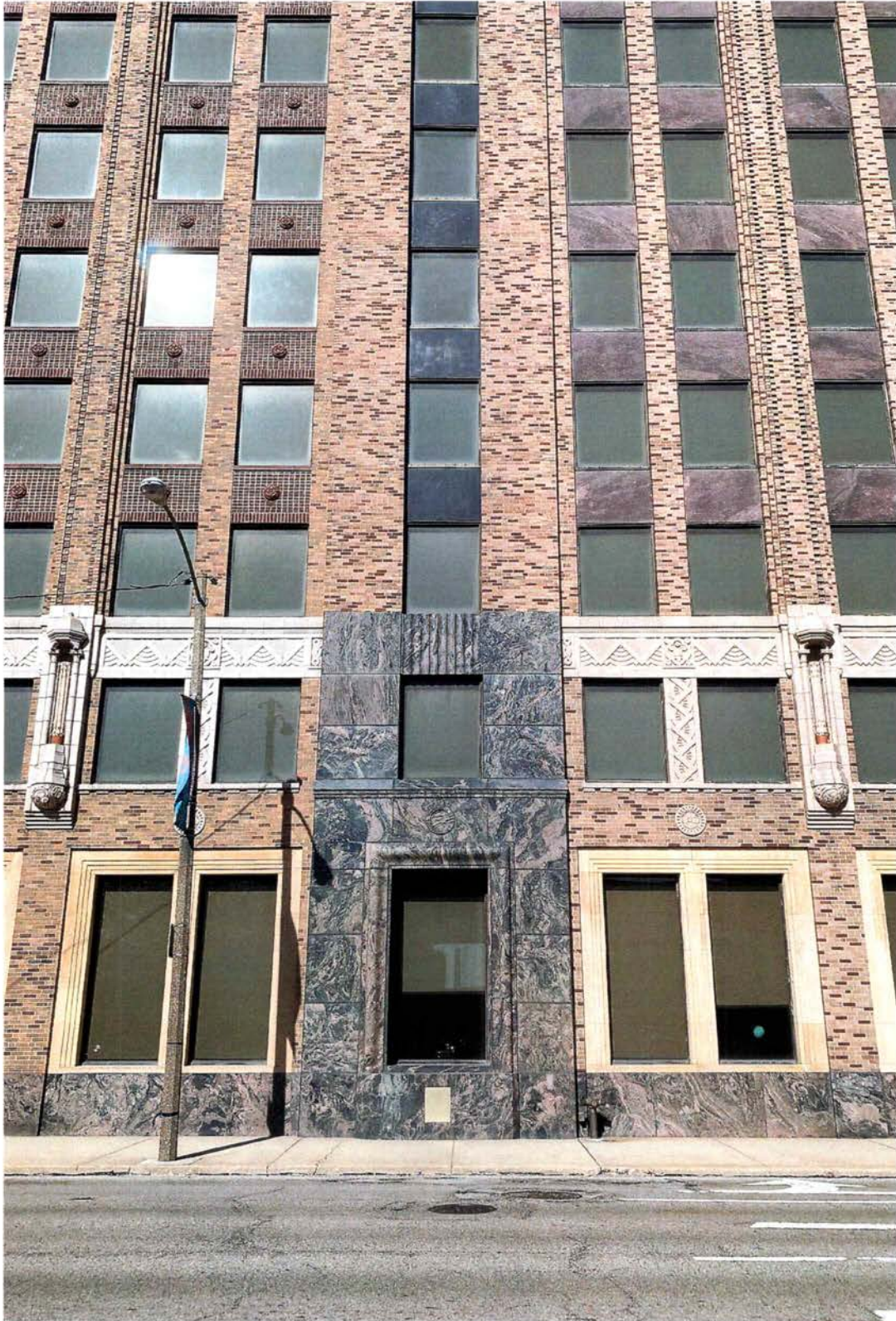
8. East elevation, center, looking west
