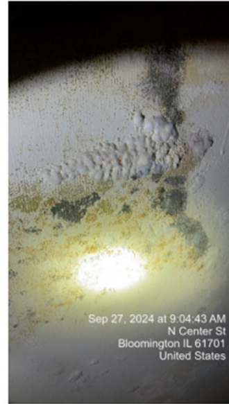
Beginning deterioration of metal components due to vacancy and lack of climate control
