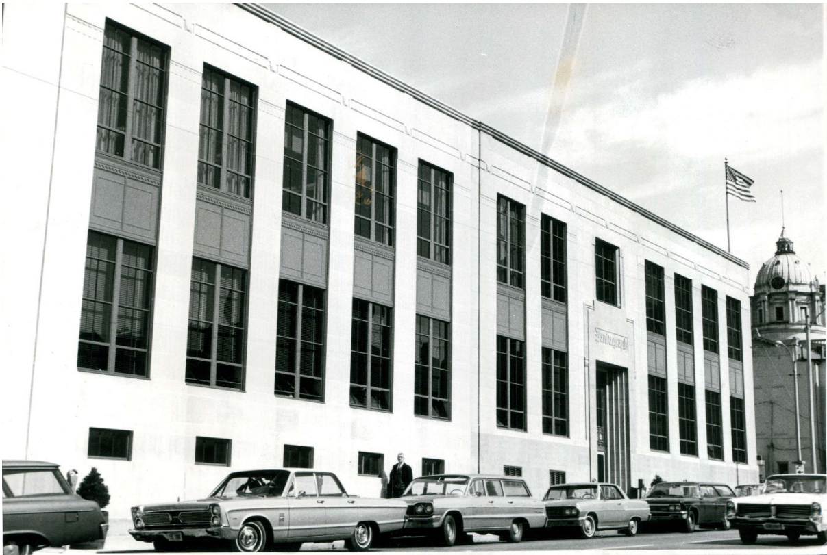
Figure 8. Pantagraph Building 1965 addition
