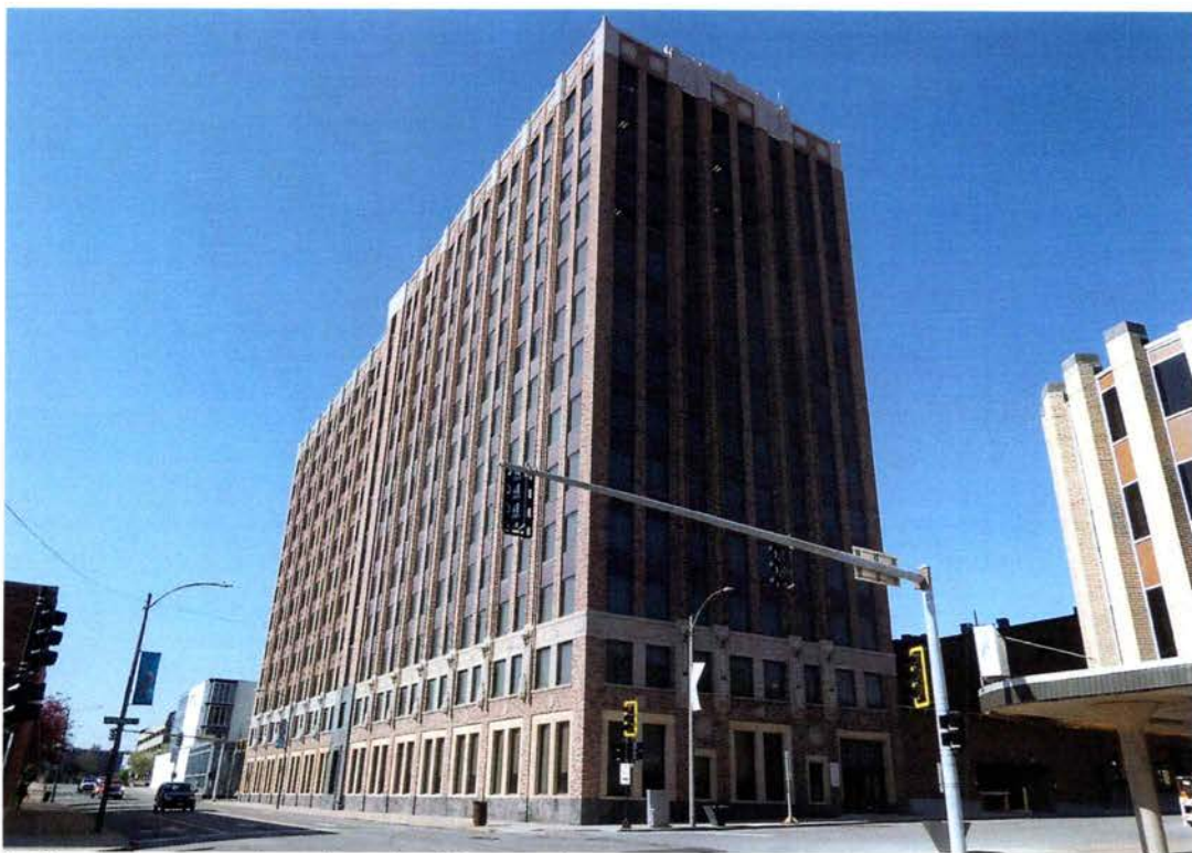
4. North and east elevations, looking southwest
