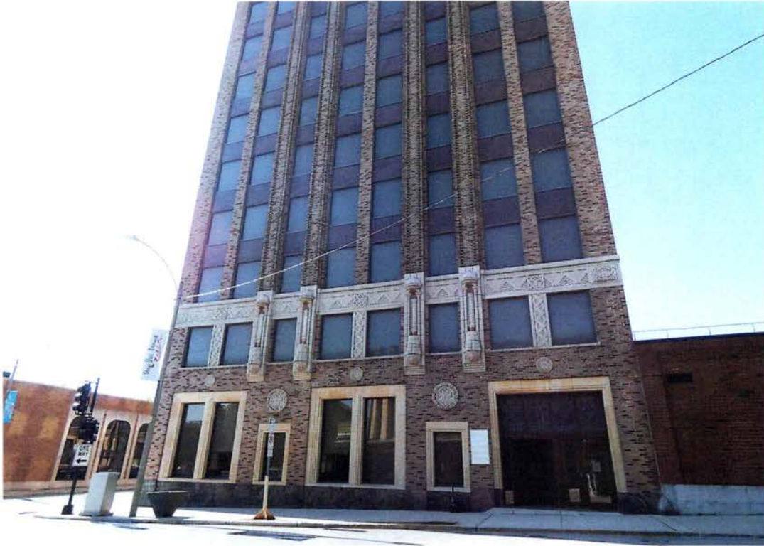
15. North elevation, lower stories, looking south
