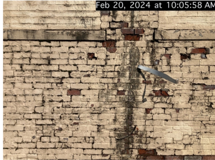
Mortar deterioration and maintenance issues on rear façade
