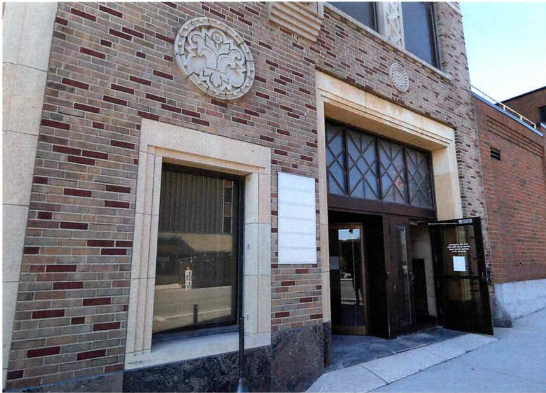
17. North elevation, looking southwest to main entrance
