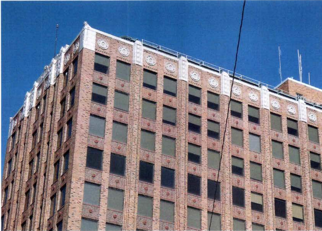
13. East elevation, south end parapet, looking northwest
