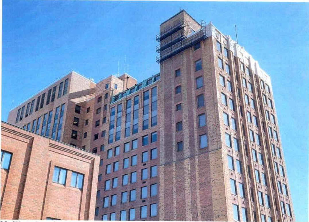
22. West elevation, upper stories, looking northeast
