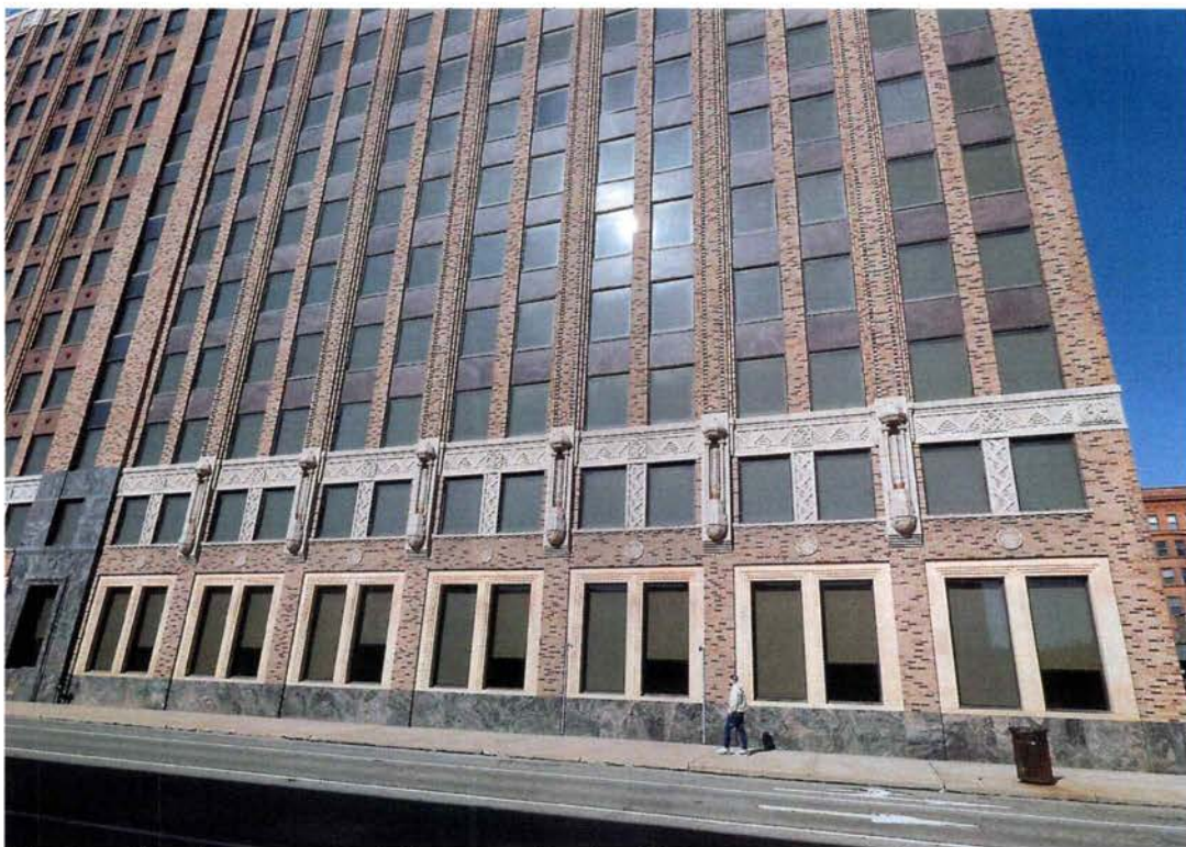
10. East elevation, north end, lower stories, looking west
