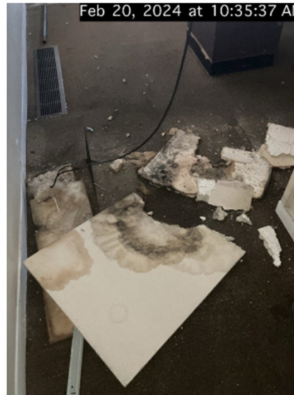
Generalized mold/mildew contamination throughout the building.
