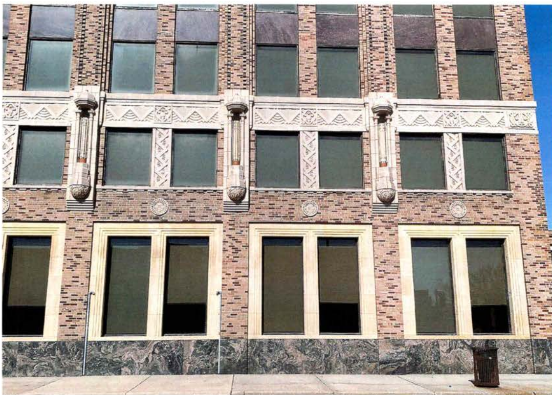
12. East elevation, north end, detail of first and second stories
