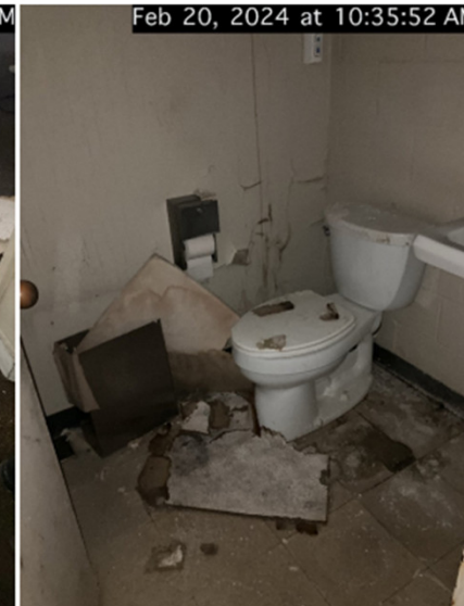
Generalized mold/mildew contamination throughout the building.
