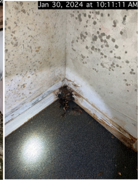
Generalized mold and fungal infestation throughout the building.
