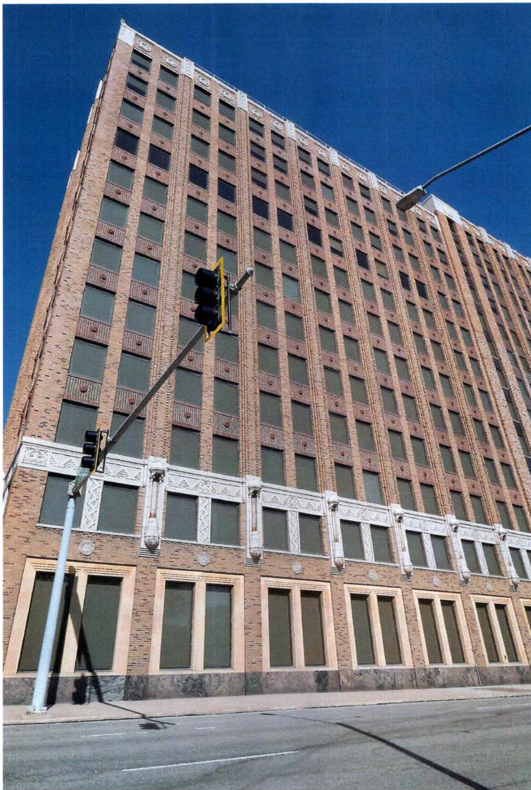
7. East elevation, south end, looking west
