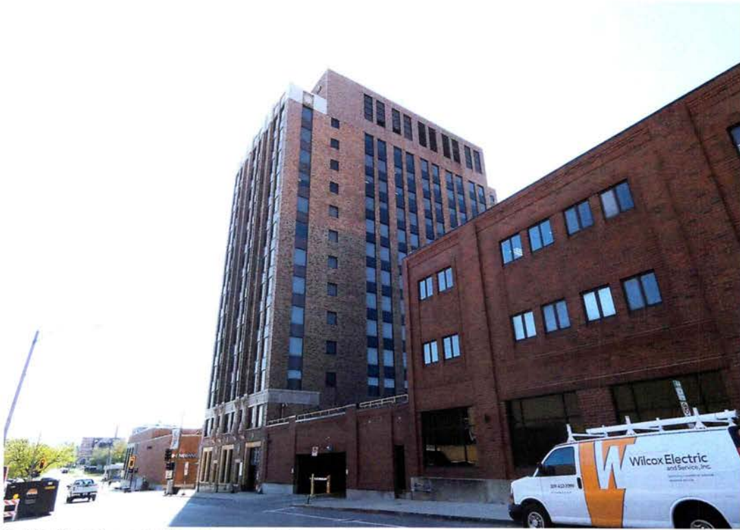
3. North and west elevations, looking east
