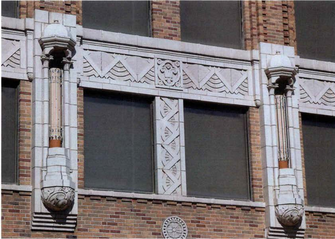
11. East elevation, detail of original light fixtures along second story
