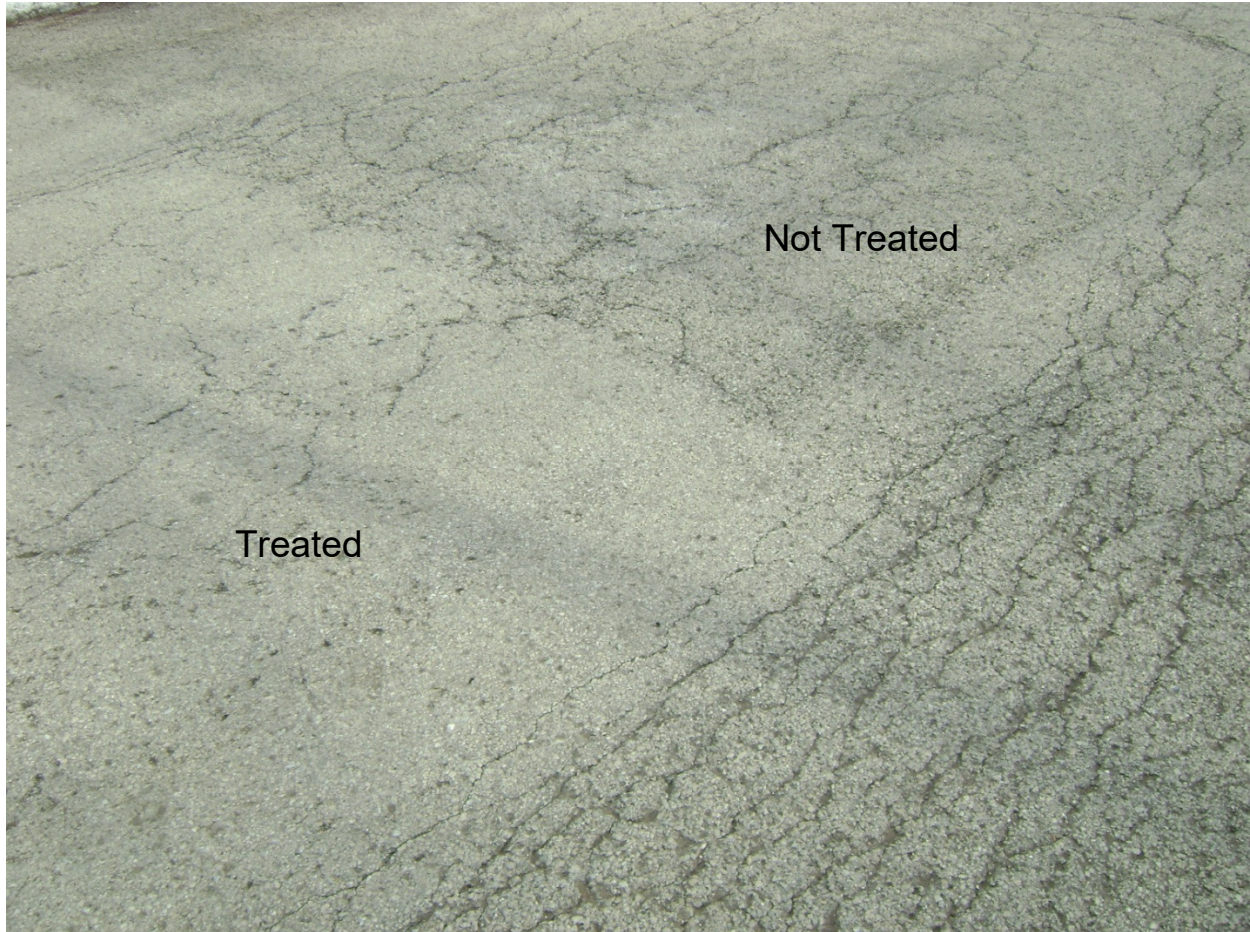
Reclamite treated asphalt pavement more than 15 years old in Yorkville, IL
