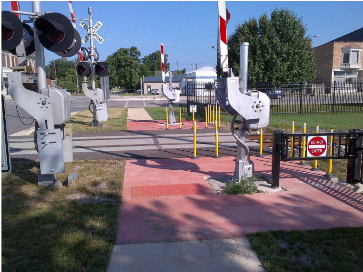
Typical pedestrian rail crossing installation
