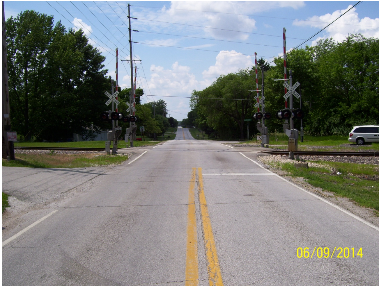
Six Pts. Rd., looking west.
