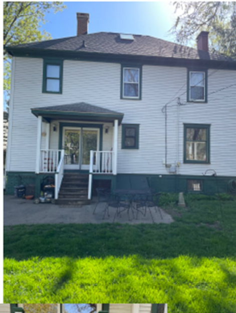
West side of home
