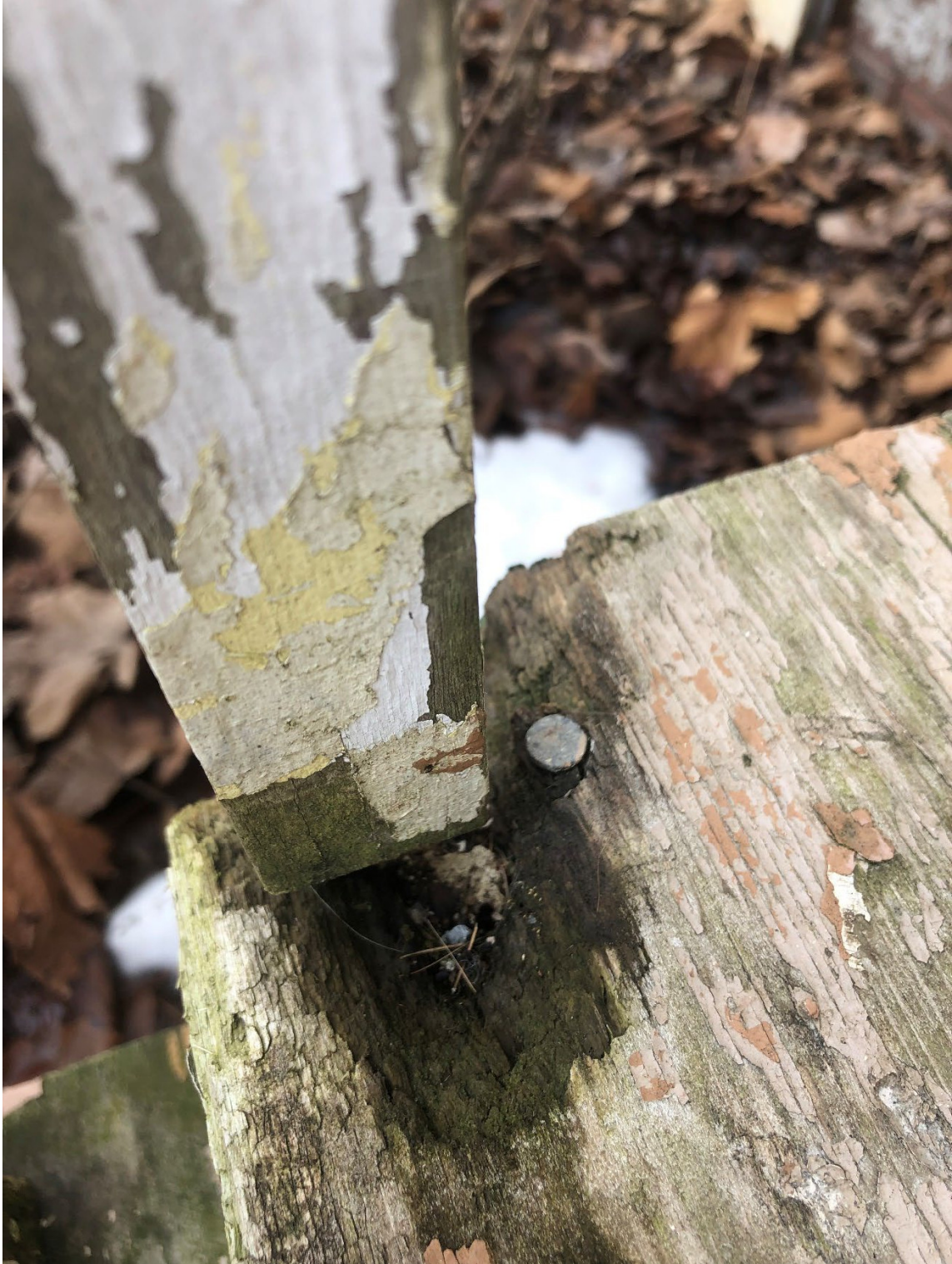
Wear on one of the steps near a spindle.
