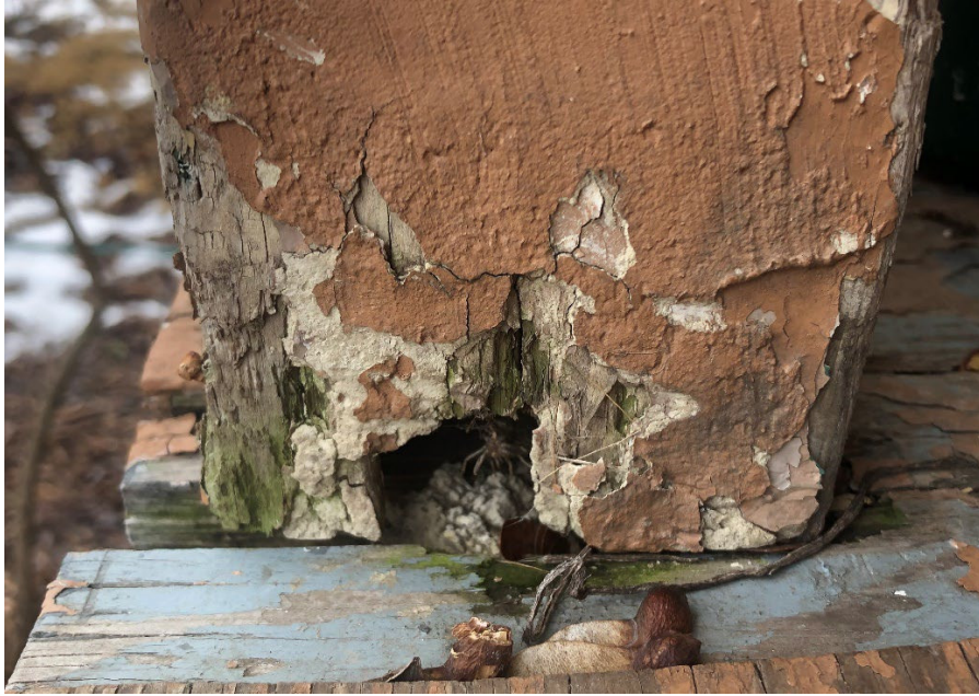
Rot to two of the columns.
