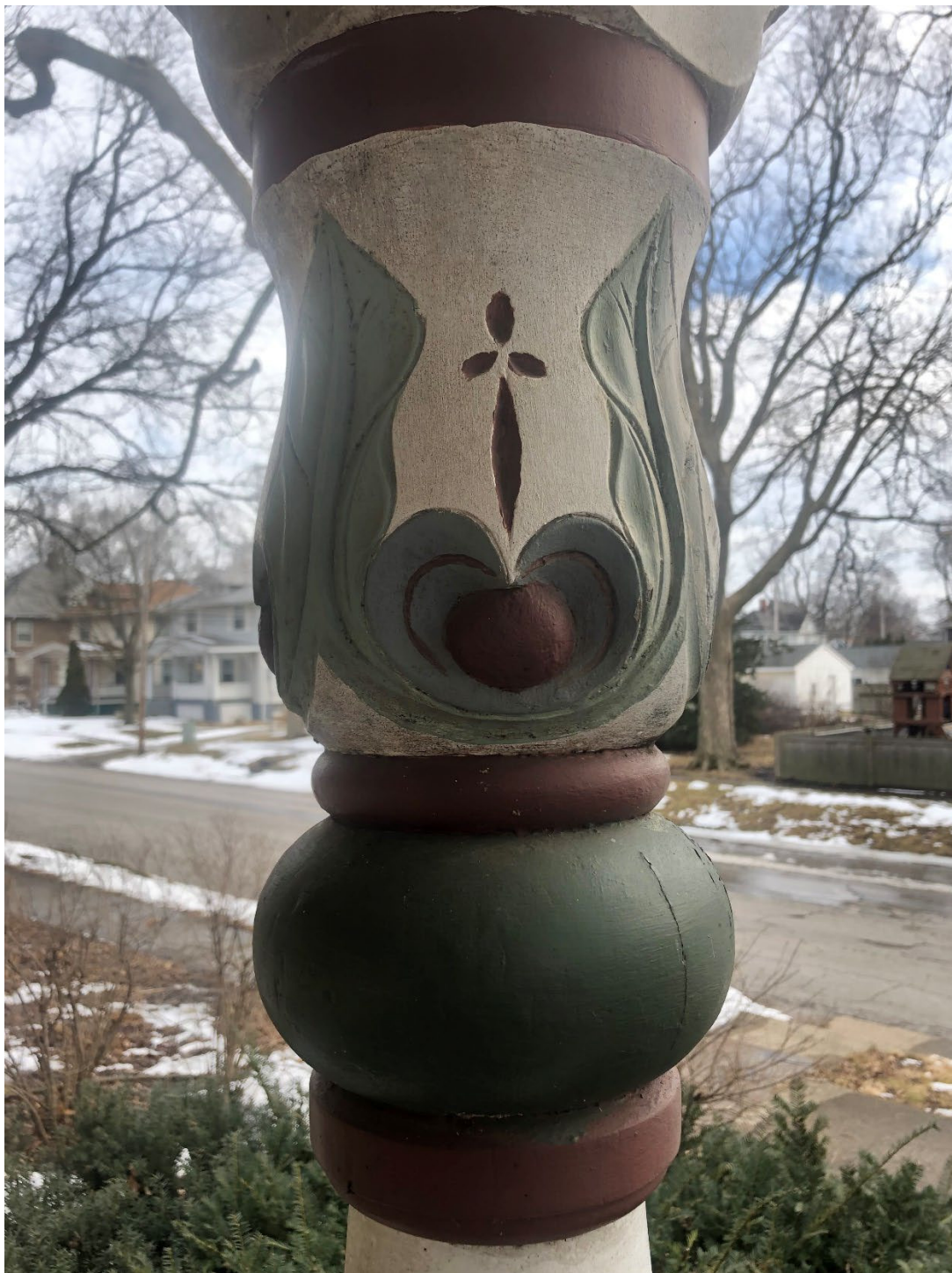
Detail of one of the porch columns.
