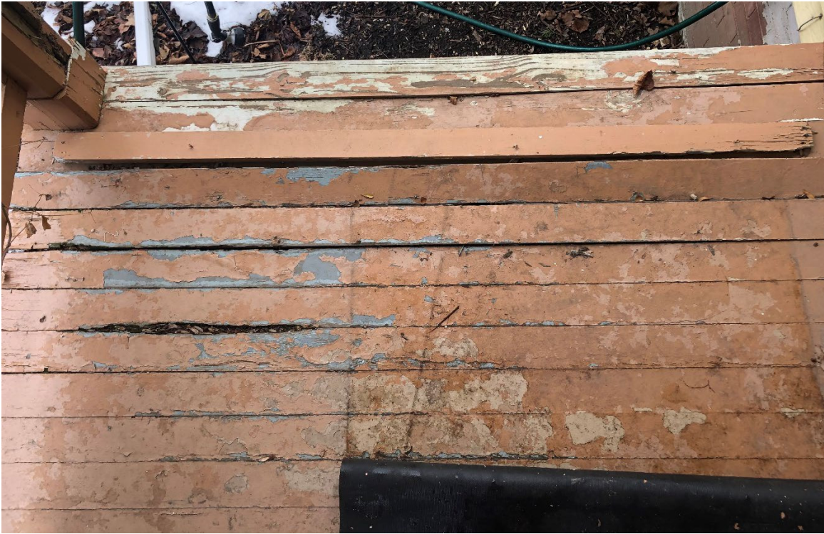
Wear and buckling to the deck boards.
