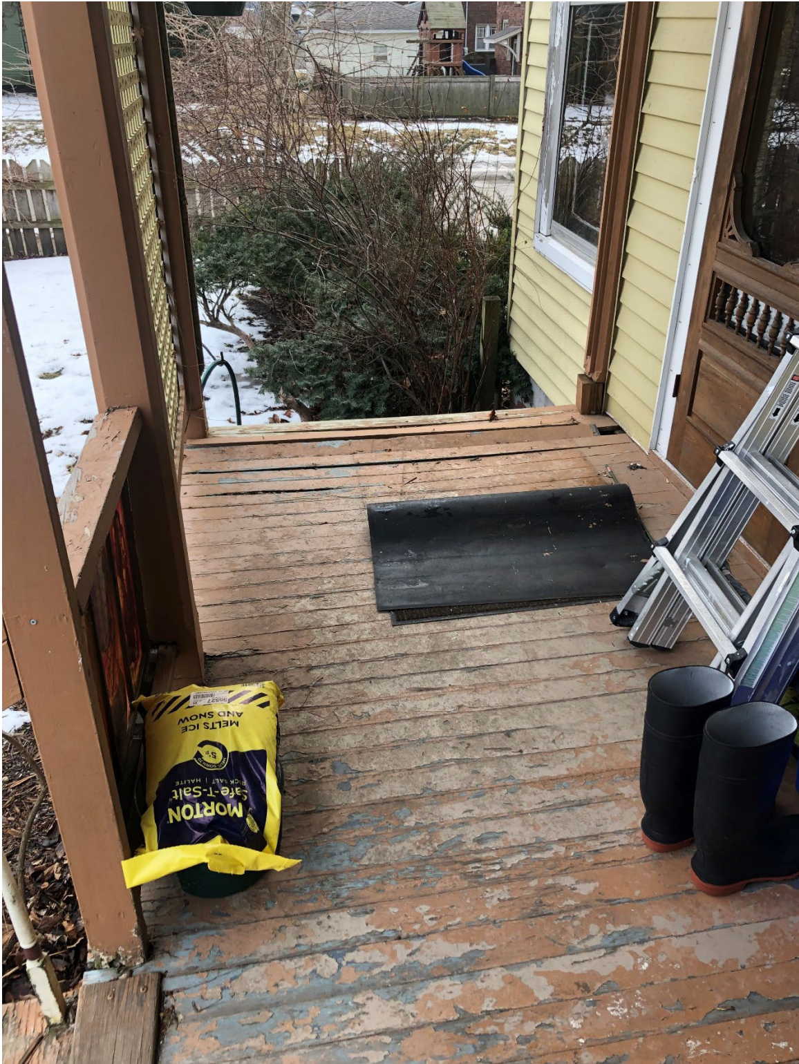
This photo partially shows the three full columns that Brad Williams believes are from an earlier structure. Buckling, wear, and old layers of paint can be seen to the deck boards.
