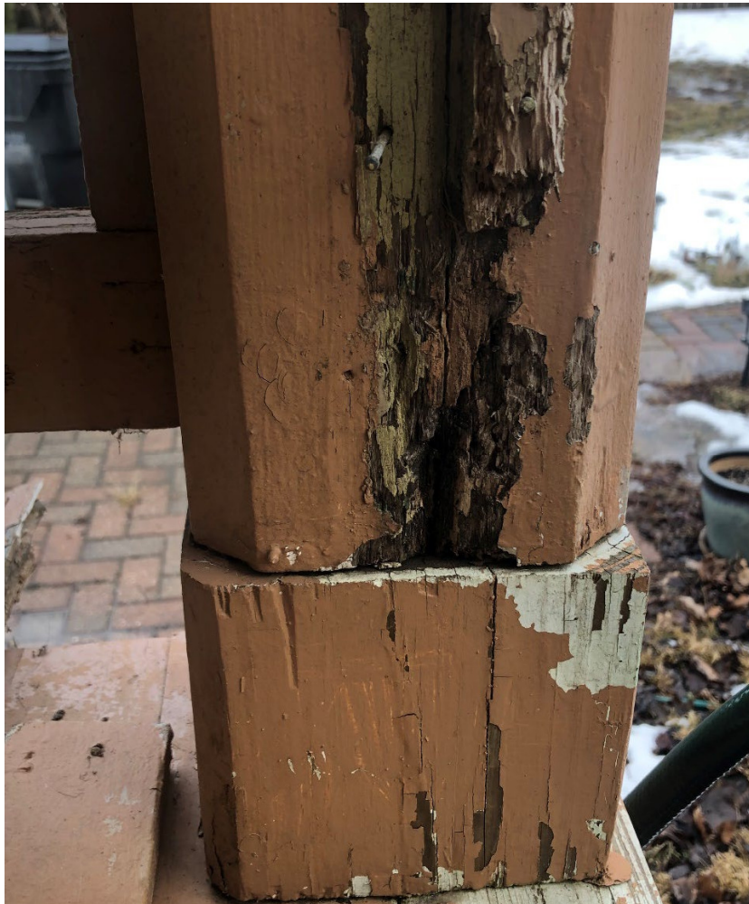
Rot to two of the columns.
