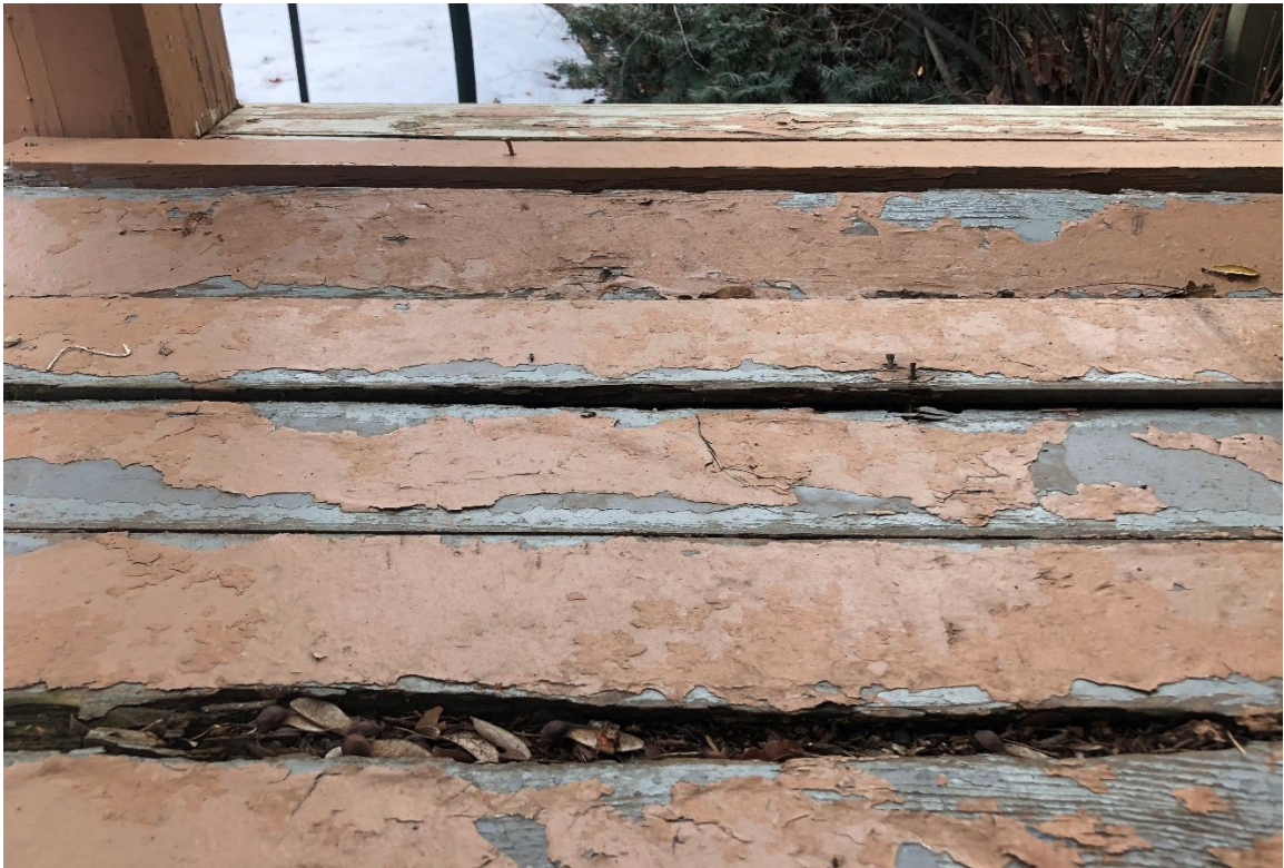
Wear and buckling to the deck boards.
