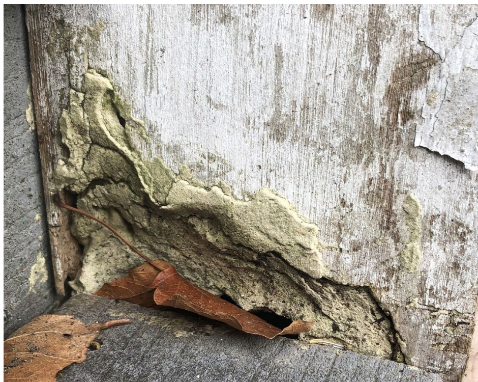
Rot at the base of one of the posts. An unsuccessful attempt at patching can be seen.
