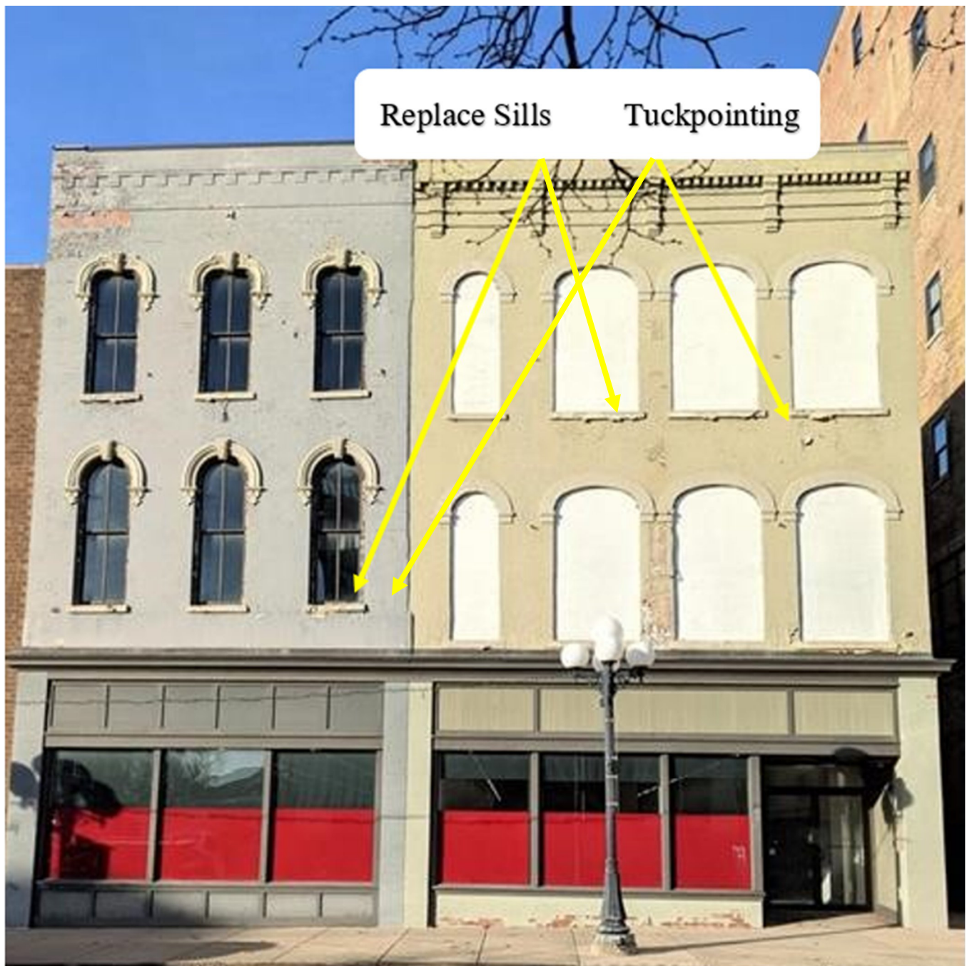
Attachment 1 - Pictures of work area (Front work area)
