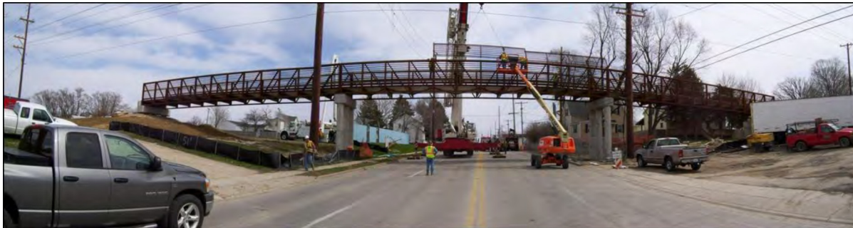
Figure 4.1. Constitution Trail bridge over Oakland Avenue.
