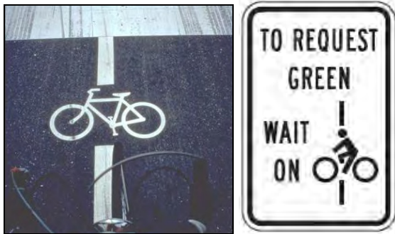
Figure 2.12. Signal activation marking and sign.
