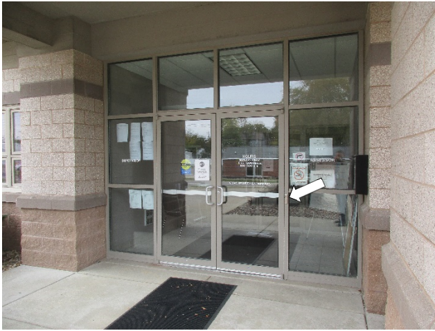
Figure 5: Door actuator
