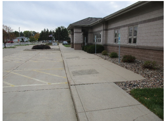
Figure 8: Curb ramps at accessible parking stalls
