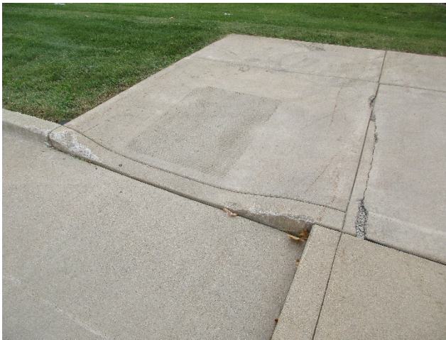
Figure 7: North curb ramp
