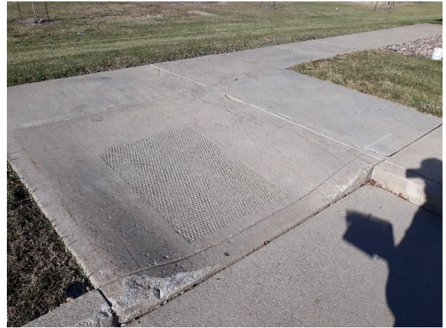
Figure 6: South curb ramp
