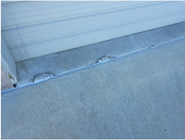
Figure 17: Concrete floor edge at Garage doors
