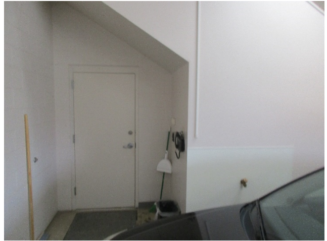
Figure 18: Swing door at Garage 129
