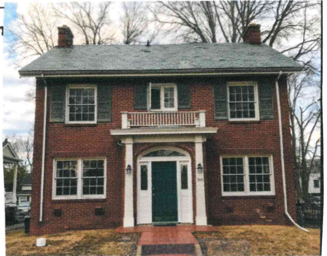
Picture of restored walkway
