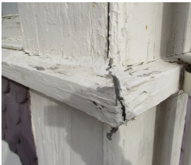
Wear and seam separation at the lower left corner area of home by the front picture window
