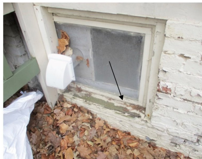
Wood frames on the basement windows around the home are in need of scraping/painting
