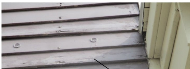
Wear and seam separation at the lower left corner area of home by the front picture window
