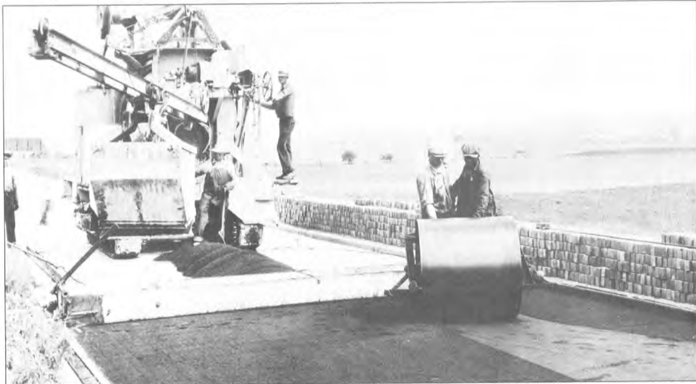
Above: Workers prepare the foundation for a brick pavement in rural McLean County about 1925. Photo: McLean County Historical Society. Below: The November 1916 Issue of Dependable Highways featured a crew setting bricks on a prepared foundation.
