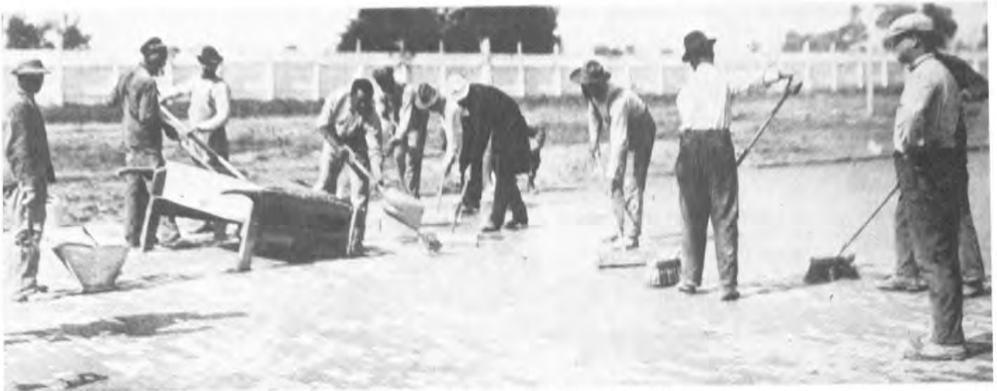
Installation of a wet cement-sand filler. Brooms and squeegees are used to fill the joints and clean the surface of the brick. This photograph appeared in Dependable Highways.
