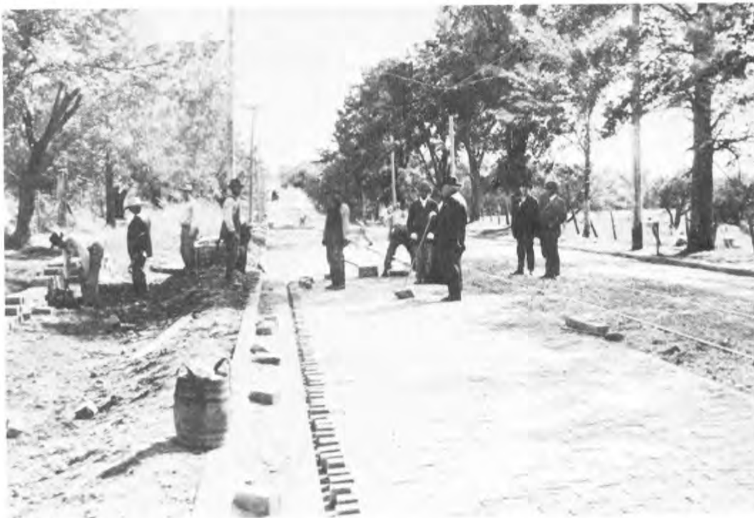
The last step in laying a brick pavement, shown in Dependable Highways, is setting the cut bricks at the curb. There, bricks are custom-cut to fit the gap. These workers are constructing the Lincoln Highway in Dixon.
