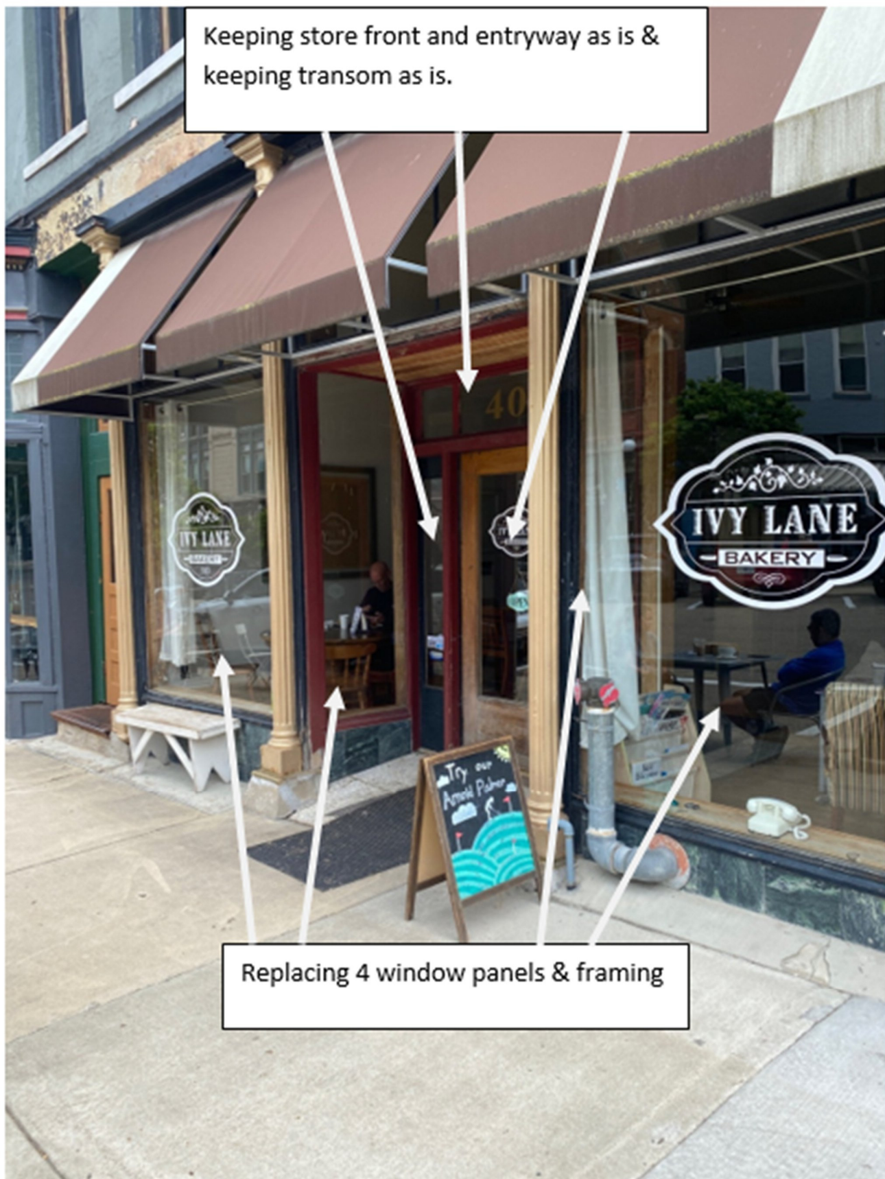
Attachment 1: Picture of Work Area
