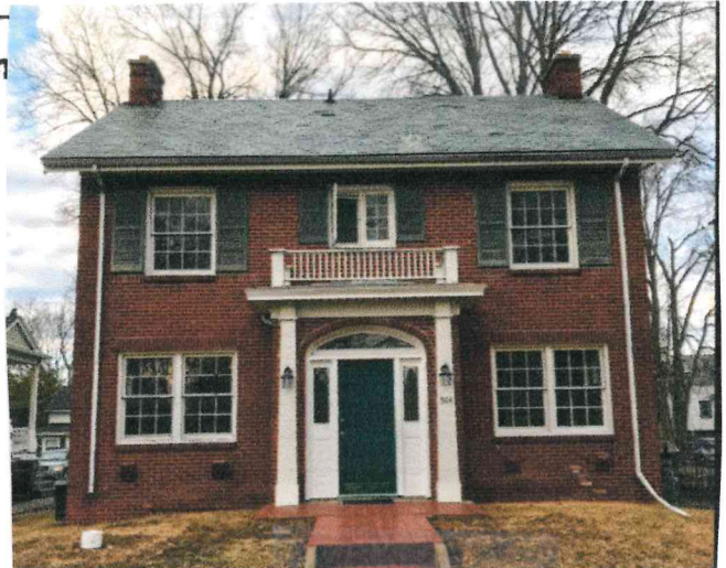
Picture of restored walkway
