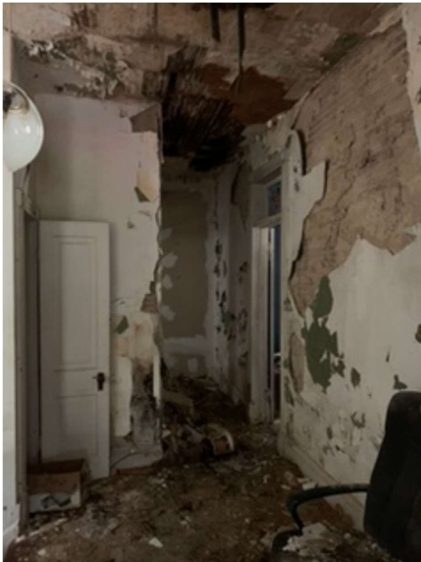
Interior damage due to roof condition
