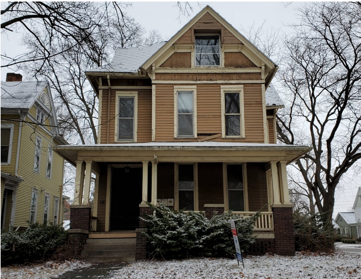
Above: The subject property at 905 E. Jefferson Street
