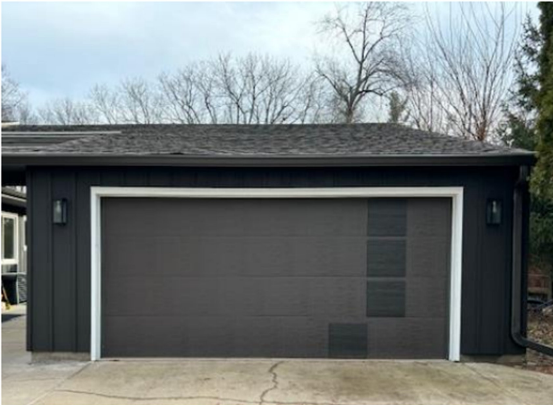
Existing 15' wide garage door
