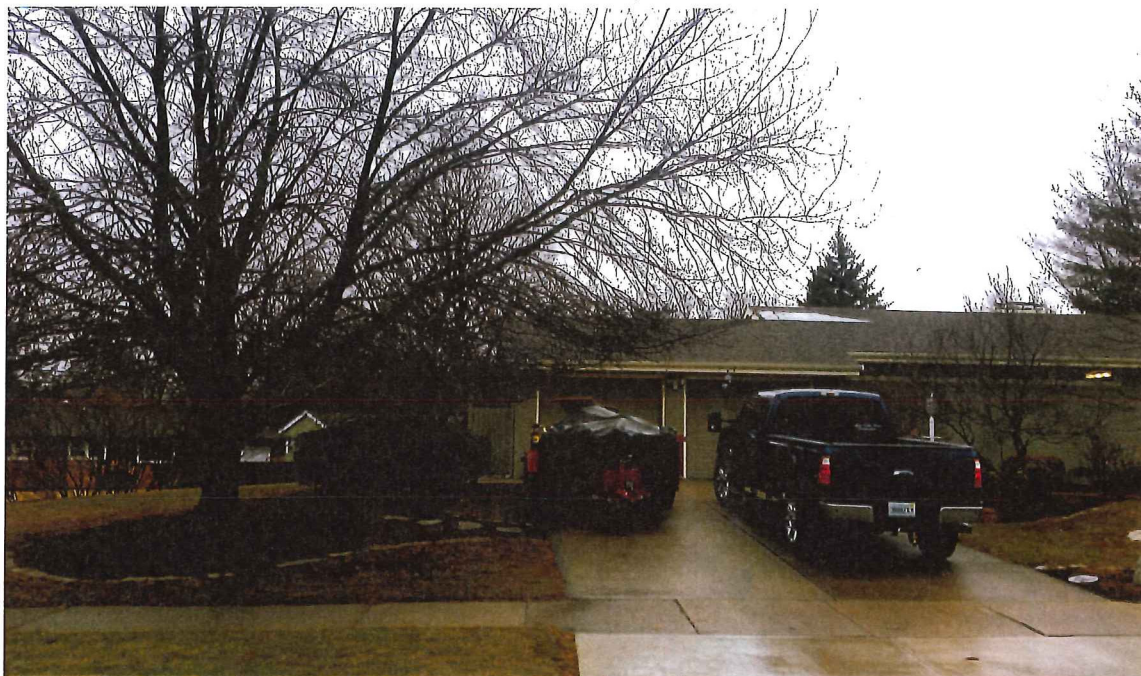
EXISTING GARAGE AND HOUSE
