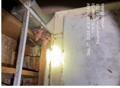
Beginning deterioration of metal components due to vacancy and lack of climate control
