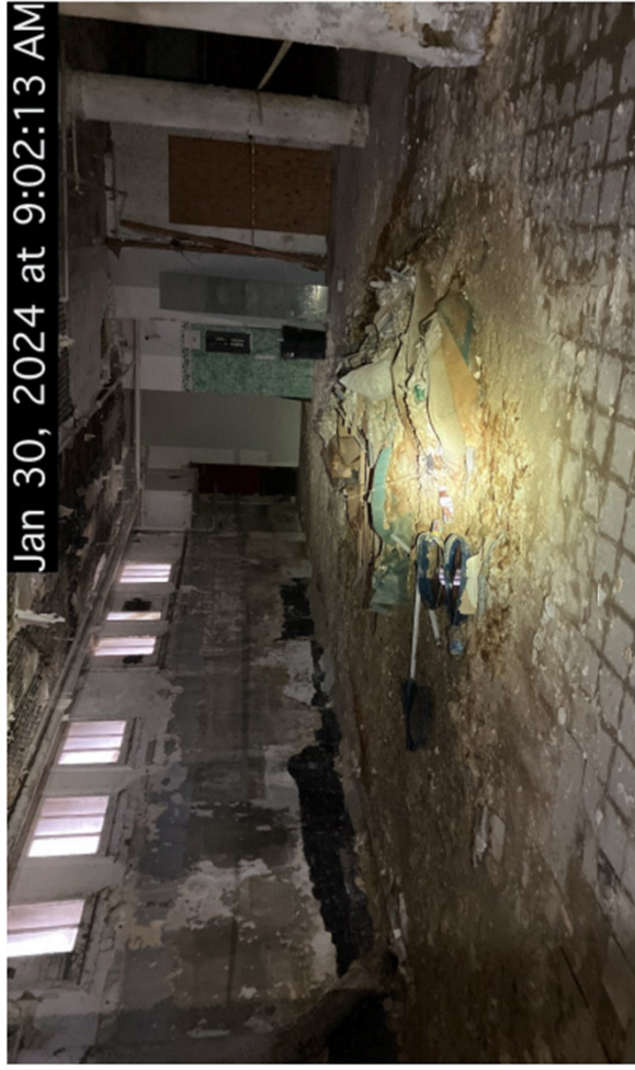
Generalized deterioration and evidence of water infiltration issues
