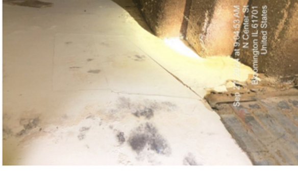
Beginning deterioration of metal components due to vacancy and lack of climate control
