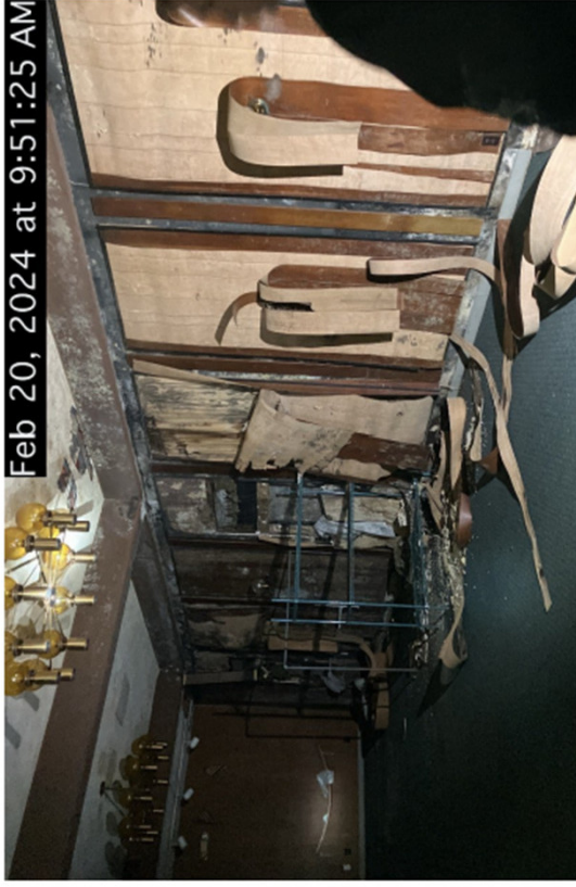
Water damage (including at least some identified structural damage)
