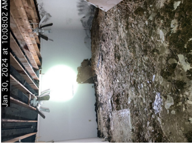
Generalized mold and fungal infestation throughout the building.
