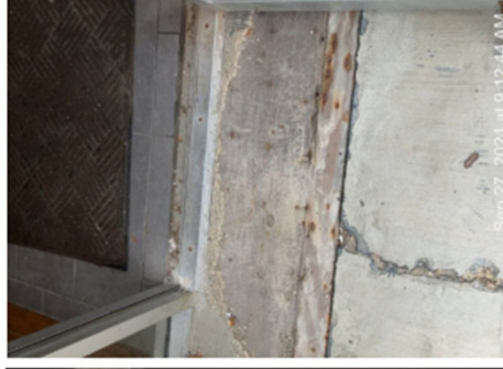
Beginning deterioration of metal components due to vacancy and lack of climate control
