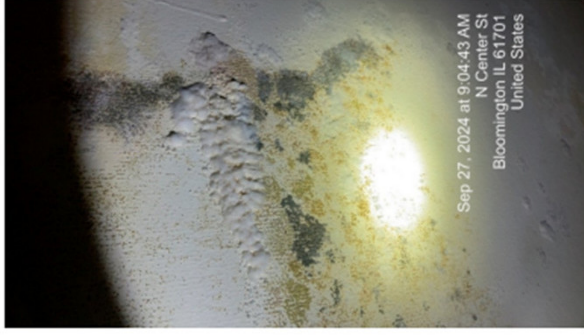
Beginning deterioration of metal components due to vacancy and lack of climate control
